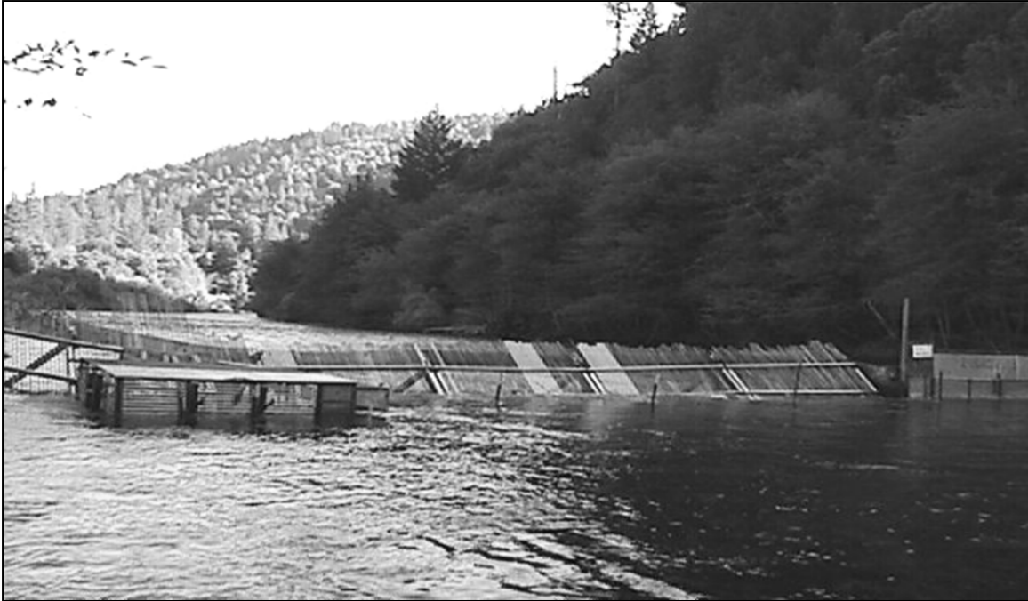
Figure 4. Typical Junction City weir configuration (looking downstream). Note the single trap box (on left) and boat gate (on right).
