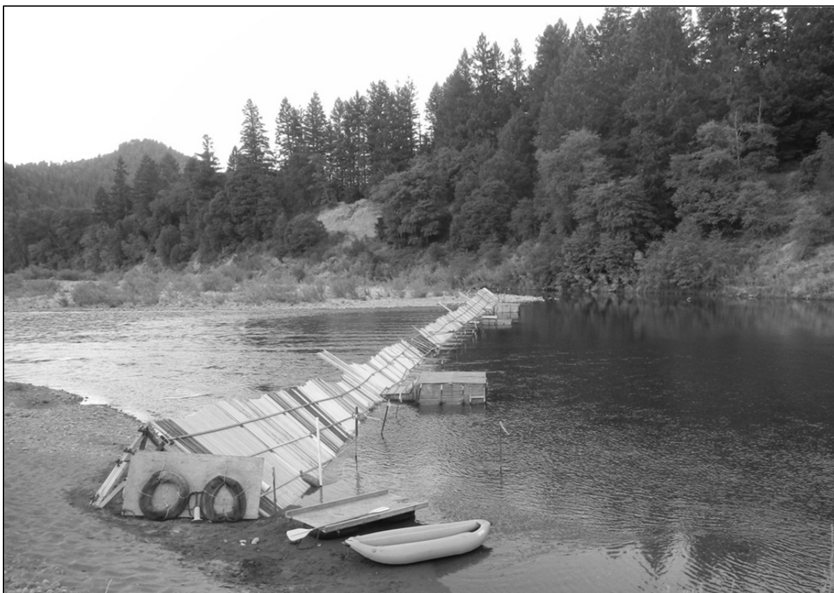
Figure 3. Set up of Willow Creek weir, 2012. Note the boat gate and three trap boxes.
