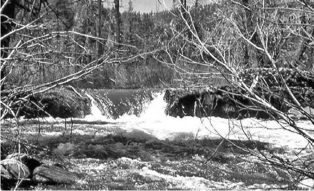
Figure 15 - Schaeffer Barrier showing collapsed center section. Circa 1999. Photo by Christy McGuire.
