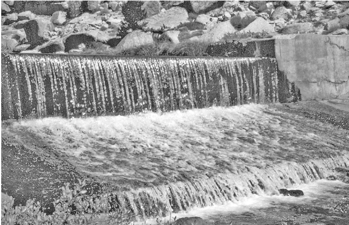
Figure 14 - Templeton Barrier following 1996 construction. October 1996.
