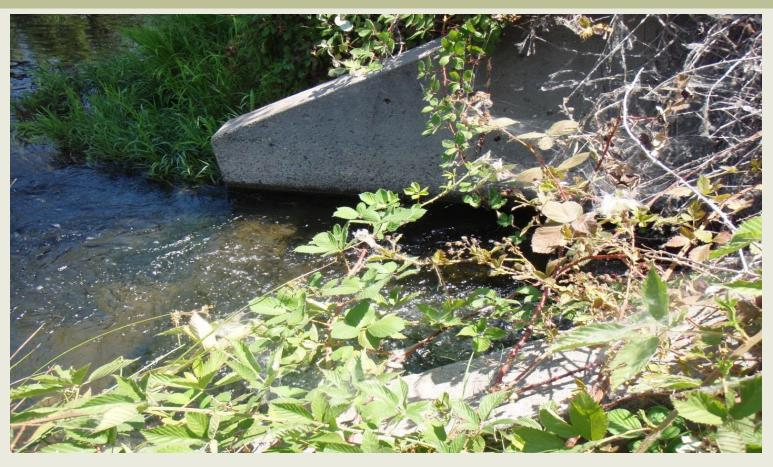
Existing storm drain outfall in secondary channel of the San Joaquin River
