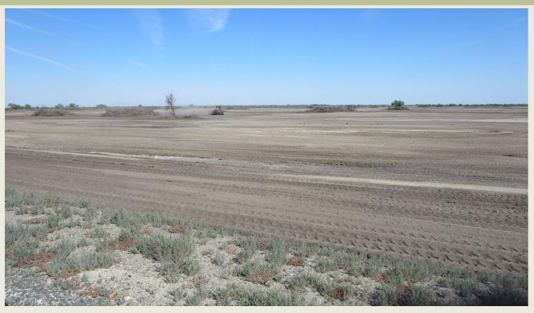
Salt Cedar removal coupled with earthwork leveling and installation of swales to enhance drainage
