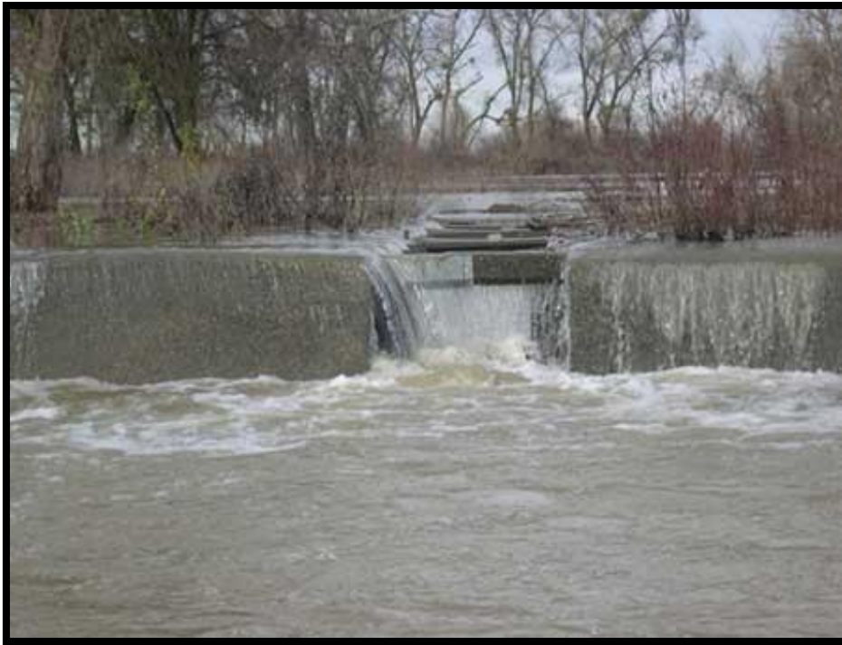
Figure 4. View of Fremont Weir Denil fish ladder during overtopping event in January 2006. Flash boards are left in place until overtopping of the weir ceases.
