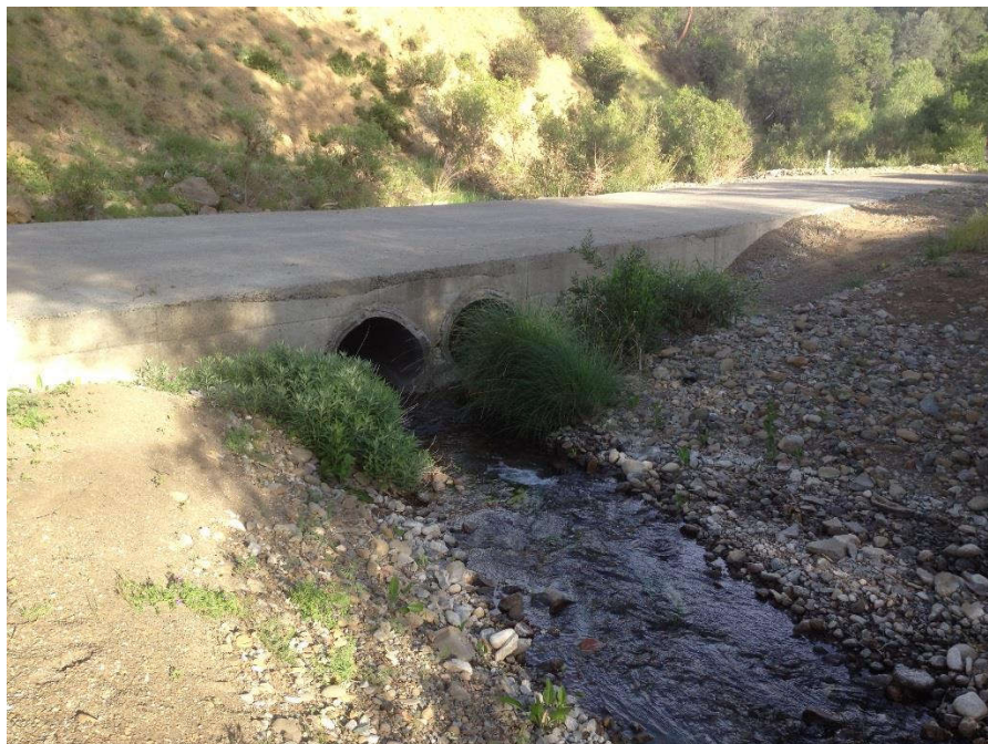
The upstream ends of the Crossing 3 RCP culverts are broken and rebar is exposed.
