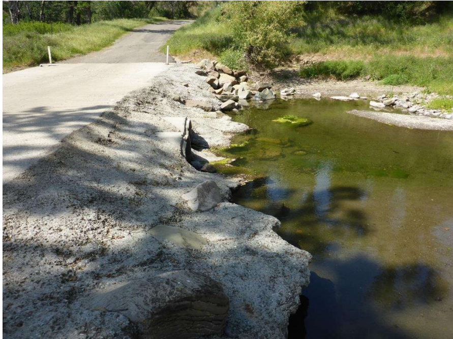
Downstream side of Crossing 1 has previously been protected with rock and gunite; however, the gunite is undermined and should be replaced with rock scour protection.
