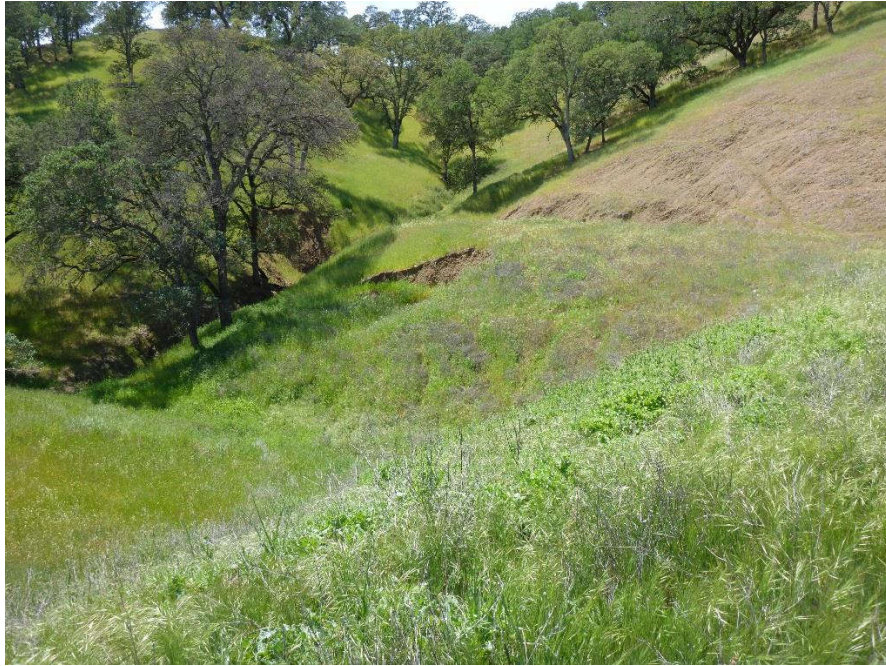
Pond P68 has erosion of the spillway embankment.
