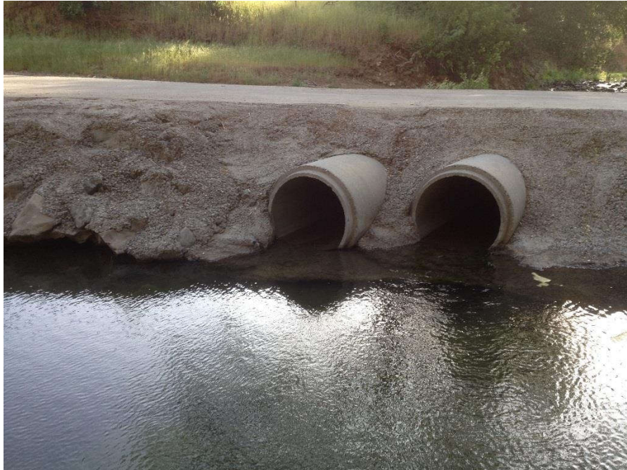
Downstream side of Crossing 3 has previously been protected with rock and gunite; however, the gunite is undermined and should be replaced with rock scour protection.
