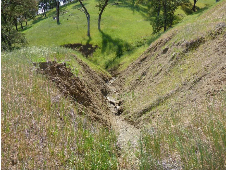
Pond P68 has severe erosion of the spillway looking downstream.
