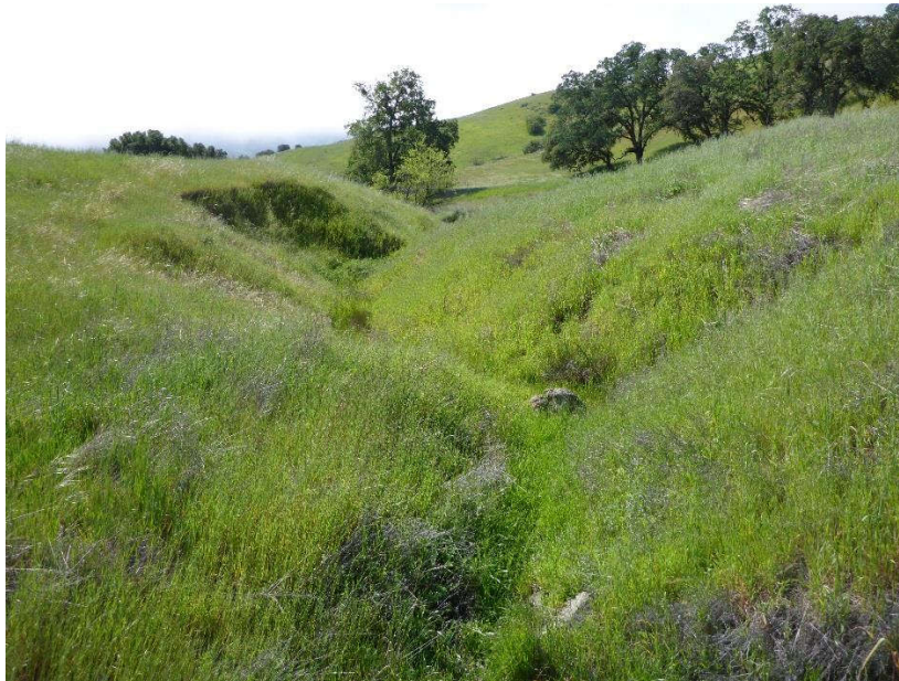
The channel at the toe of the dam is eroding.
