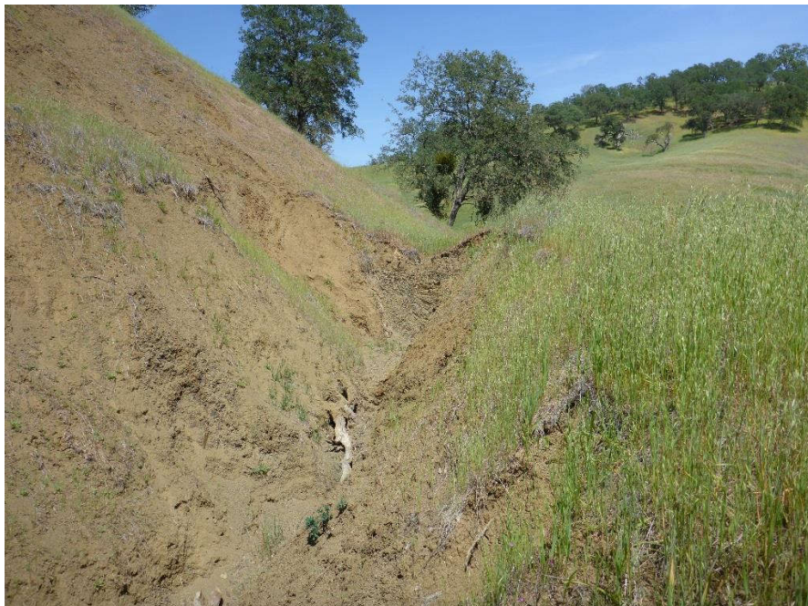
Pond P68 has severe erosion of the spillway looking upstream.
