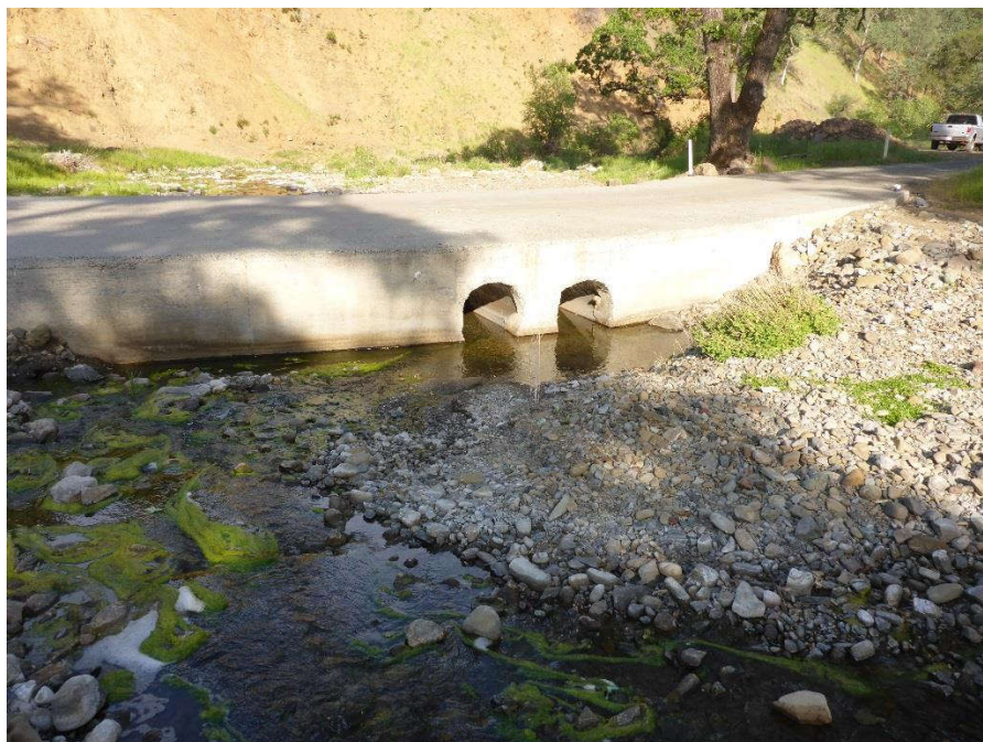
Upstream side of Crossing 1 is not undermined and has no pool.
