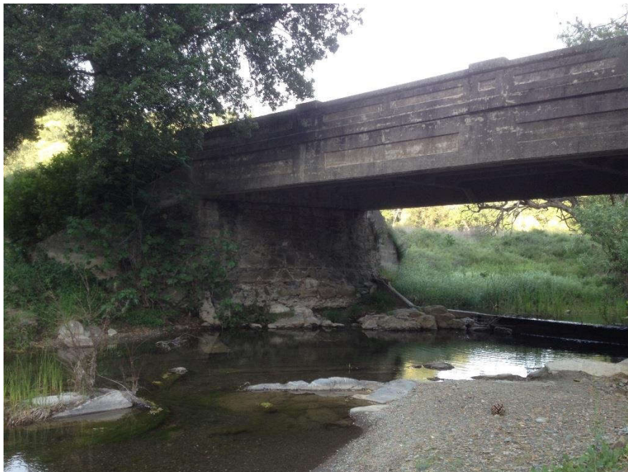
The weir between the bridge abutments restricts fish passage, and one or two notches should be cut in the weir.
