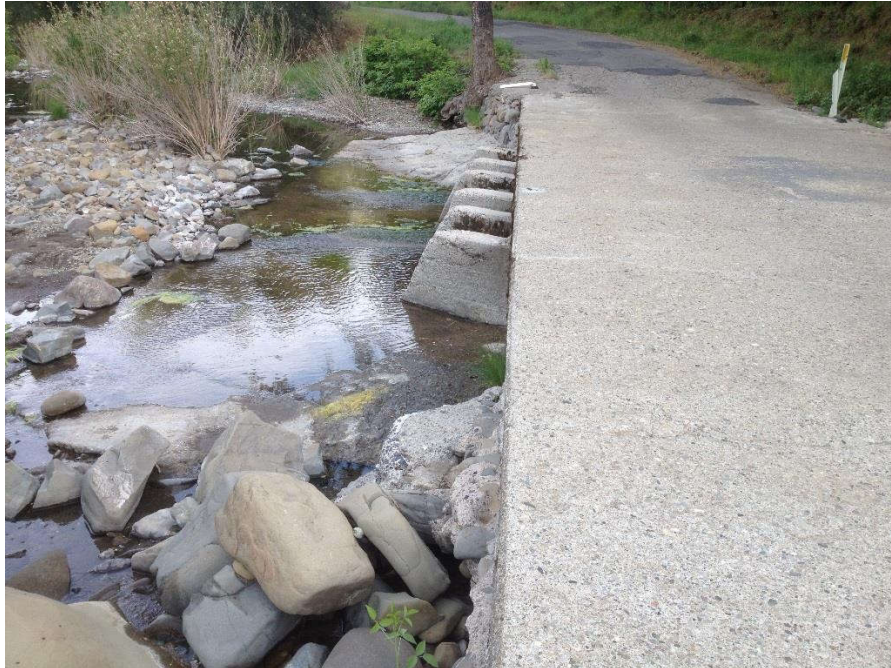
The downstream side of Crossing 5 has a concrete apron that appears to have protected the crossing from undermining.
