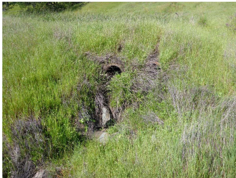
The dam embankment is eroding below the twin pipe outlet.
