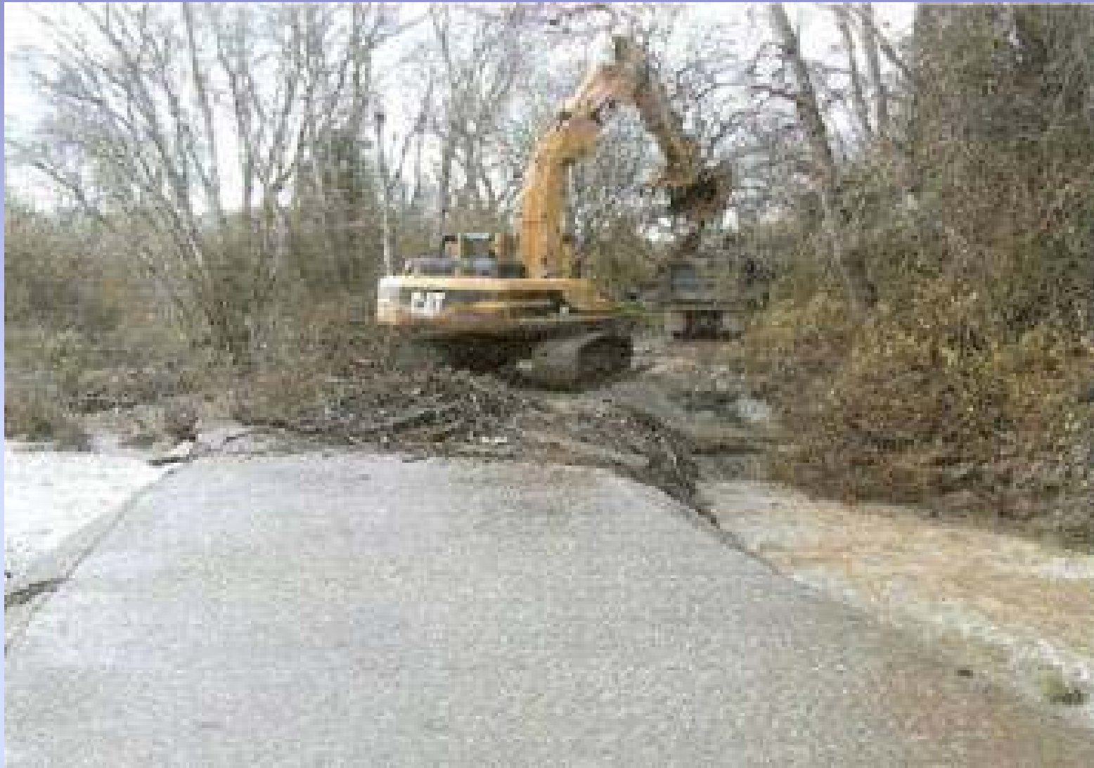
Debris accumulation on Ferrasci Road crossing
