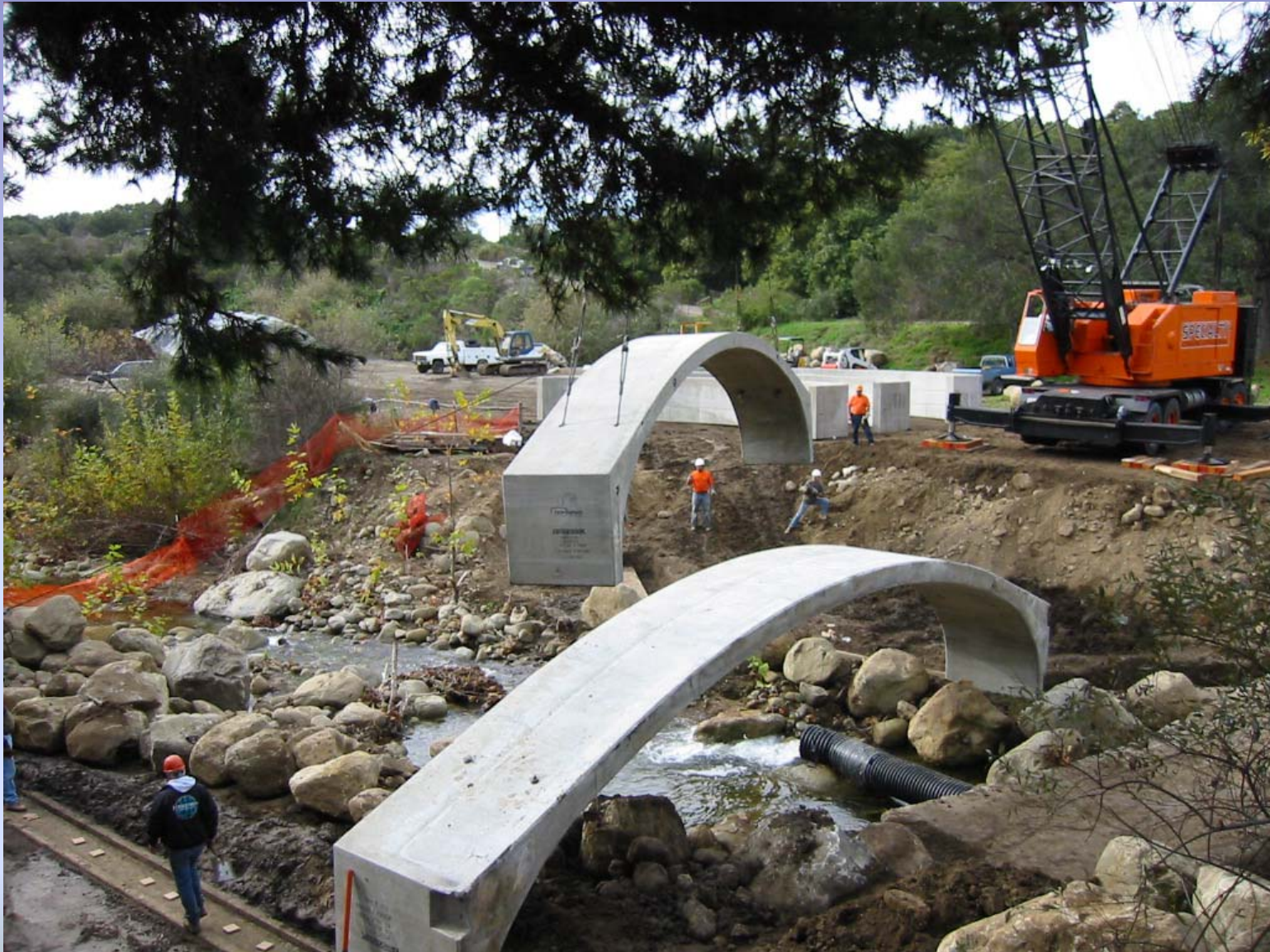
Pre-fabricated bridge installation on El Capitan Creek
