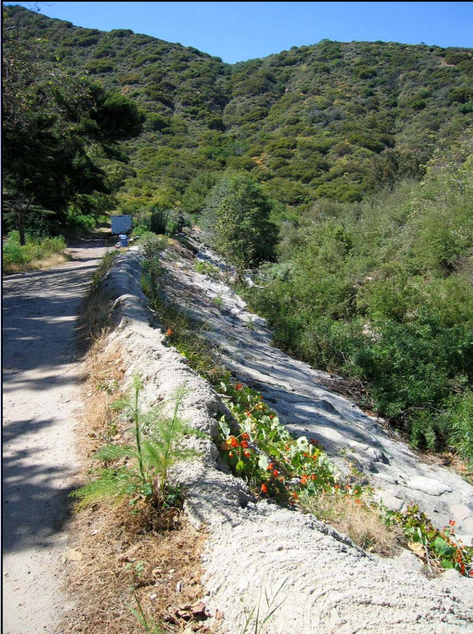
Edge of Berm showing concrete stabilization of sides
