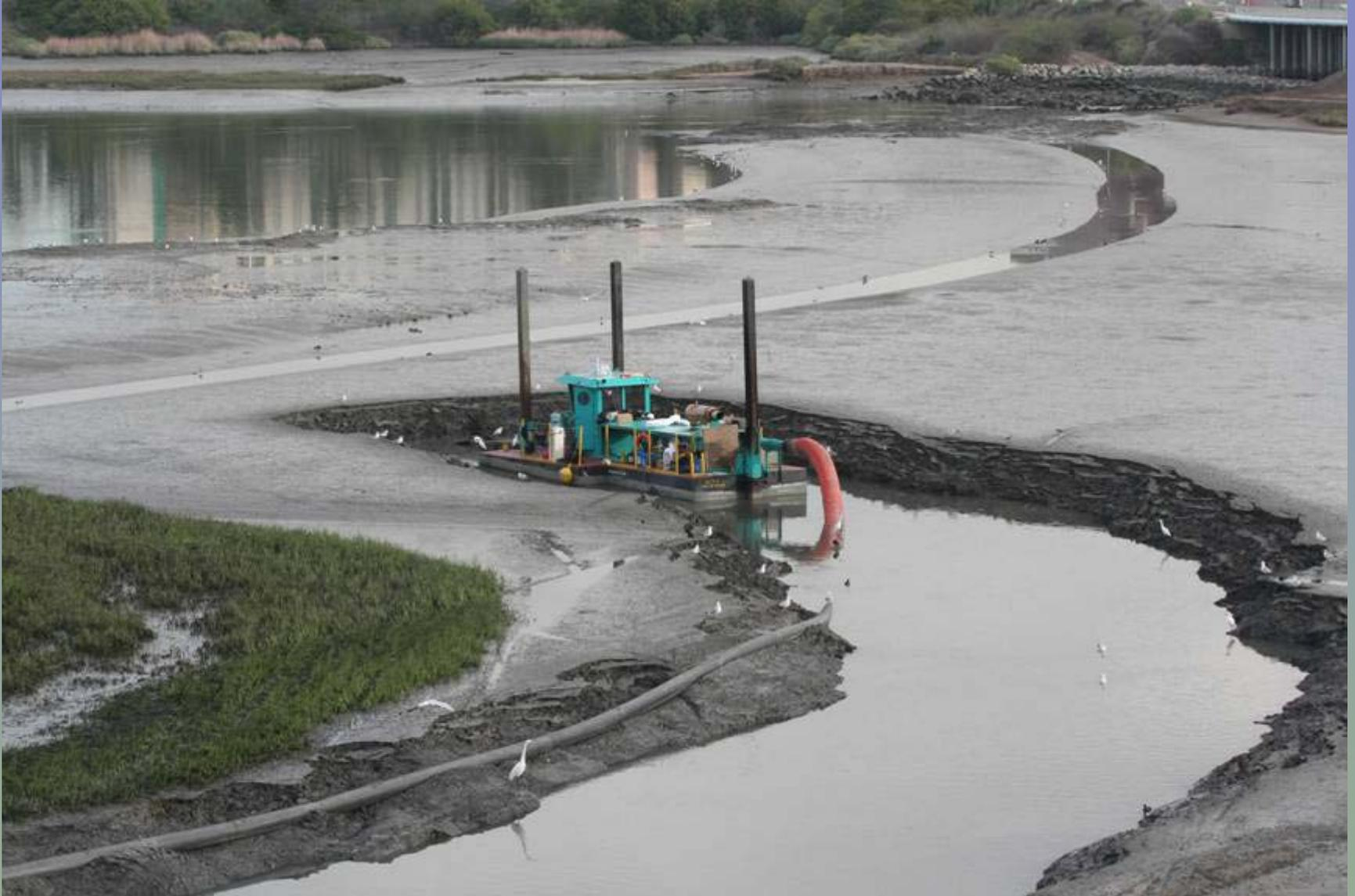
Hydraulic dredge working to deepen channel (see excavation of side walls).
