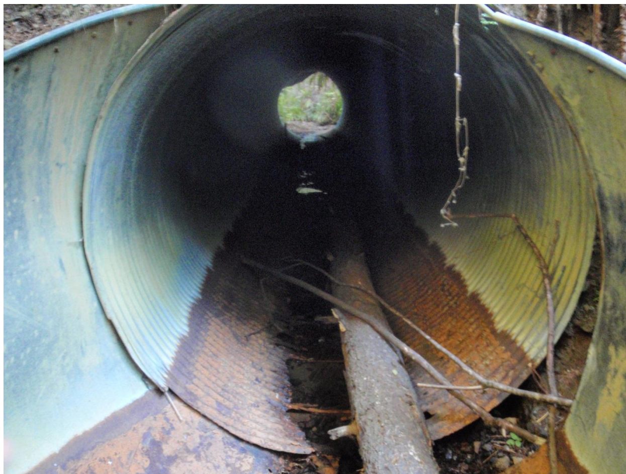
Photo 2: Habitat Unit #73, rusted culvert with a tree inside of it. Photo taken on 9/28/2016
