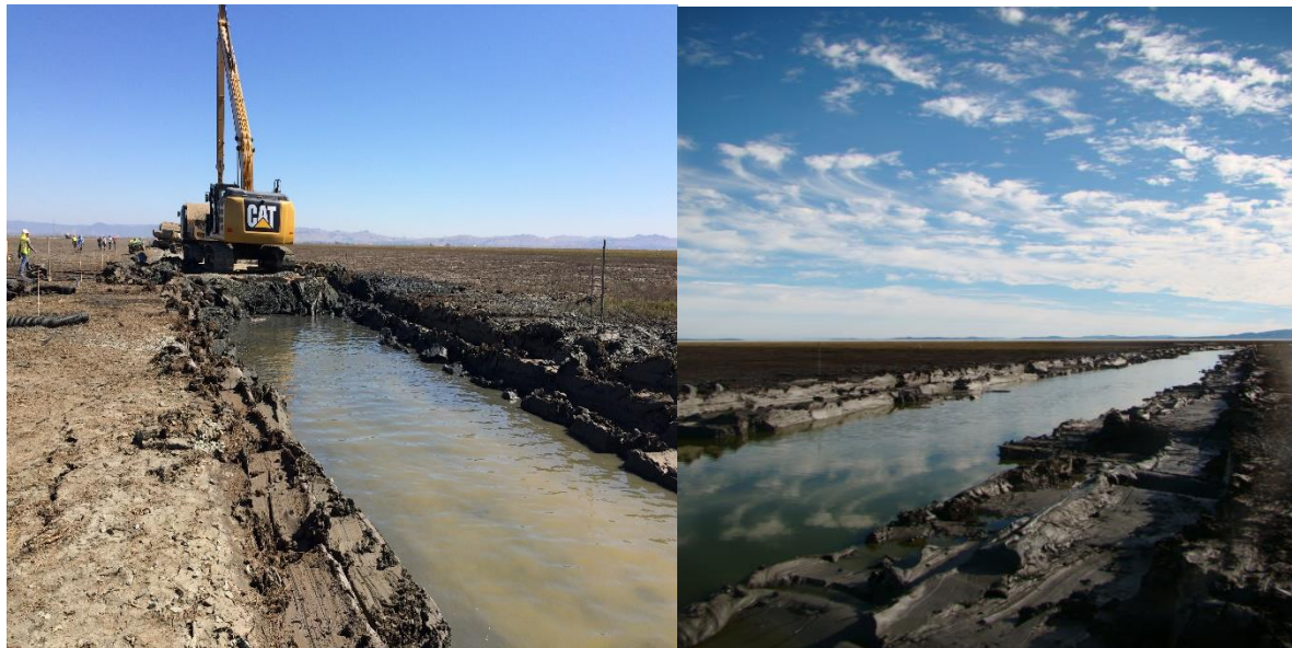
Figure 12 and 13. Show the completed excavation of the southern half of the channel, points 22+00 to 45+60. Note the stair-step/bench effect shown in figure 12 to relieve slumping pressure of unstable marsh soils. Water shown filling the channel in these images has leached from the central basin top and marsh soil, this channel is not yet open to Sonoma Creek's natural tidal flow.
