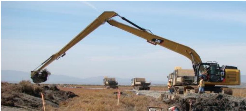
Figure 21. Marsh mounds were placed approximately 20ft from the edge of the channel, noted by wood stakes with orange tops. Mounds are expected to shrink about 50% with sun/air exposure and winter storm events and tidal flow.
