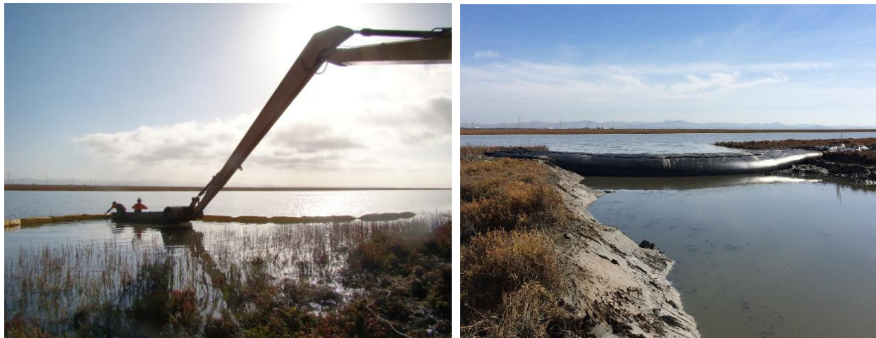
Figure 14 and 15. Connecting the northern half of SCEP channel to Sonoma Creek was a feat requiring many installments including the set-up of an exclusionary curtain, excavating the first 70 ft of channel mouth, and then the placement of a temporary Aquadam. Both the curtain and Aquadam (pictured here) prevent wildlife from entering the worksite during construction, a biological monitor was onsite for the entirety of the installation.
