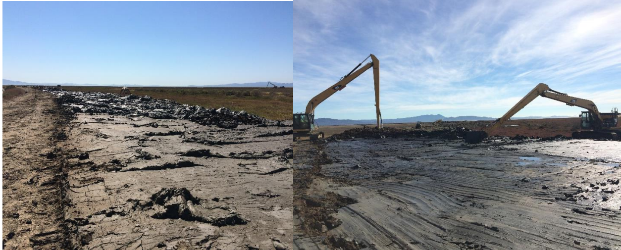
Figure 24 and 25. The left figure shows the original placement of the transition ramp's material. Material was placed as far as the excavator arm could extend from the levee on the left. The photo on the left shows the work done through Hanford's contract extension, originally proposed for 2017. With the help of a second excavator pulling from within the marsh, material is dug down 100-120ft from the levee creating a gently sloping habitat ramp which has already begun to naturally revegetate. High marsh revegetation by STRAW begins fall 2016.
