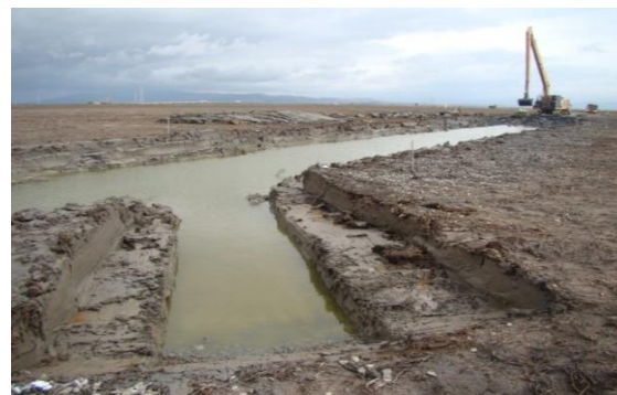
Figure 19. Seven, 20ft long lateral starter channels are expected to naturally extend into the marsh with annual tidal flow. These will be monitored for future development.
