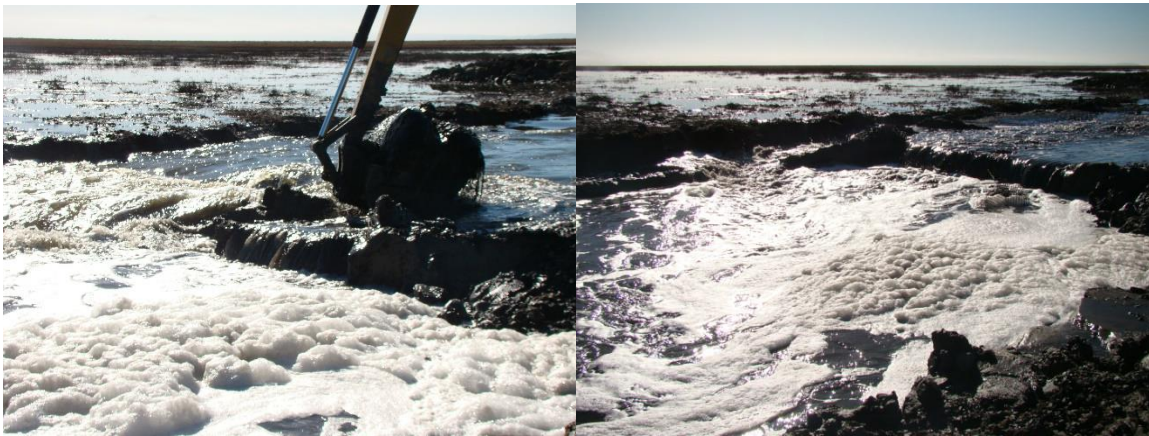
Figure 16 and 17 show the final excavation component of the channel. A 20ft soil plug was carefully removed to unite the southern and northern channel halves and allow trapped water from the central basin and southern channel half to finally flow out to Sonoma Creek. The team had to work carefully to regulate water release as the 1,000s of gallons of water could have forced through the plug, distributing the sediment into the channel and caused impediments to flow.
