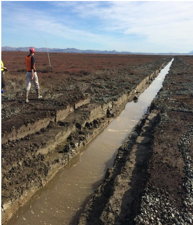
Figure 18. Staff walk along the lateral access road channel created to mitigate the depressions the weeks of heavy machinery traffic caused under the access road. This channel now stretches from the levee to the mid-way point of the main channel and ties in pre-existing MSMVCD channels to create an enhanced drainage network.
