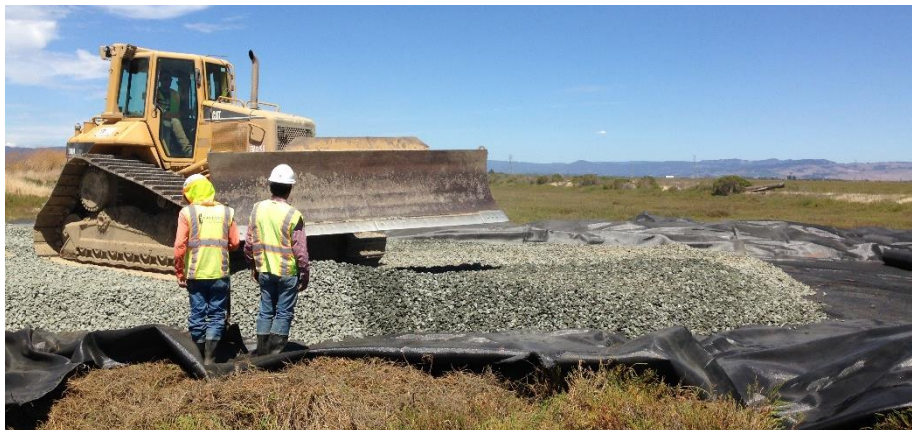
Figure 11. Hanford crew create an 18in-36in thick permeable access
