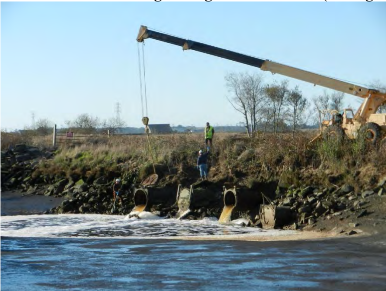
Site 19: Two of McDaniel Slough tides gates being chained open –Dec 2012 –West view
