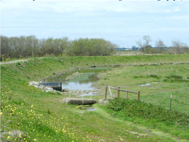
Site 18: Tide gate/drainage pipe installed in 2012 - March 2013 - Northwest view (with reconstructed City levee in background)
