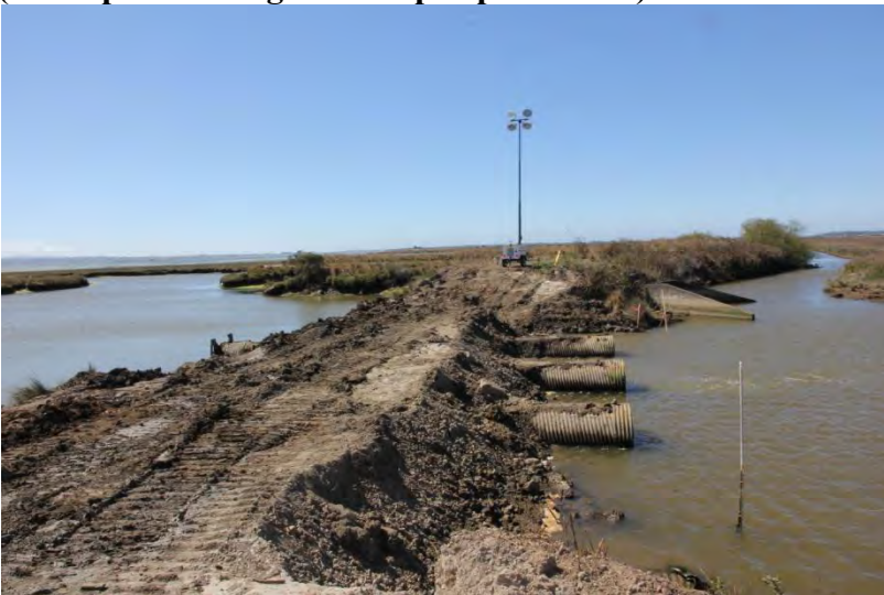
Site 19: Initial excavation for McDaniel Slough levee breach –Sept. 2013- West view
