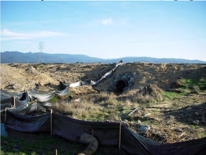
Site 6.1: CDFG culvert/tide gate installed in 2009 – Dec. 2009 – South view
