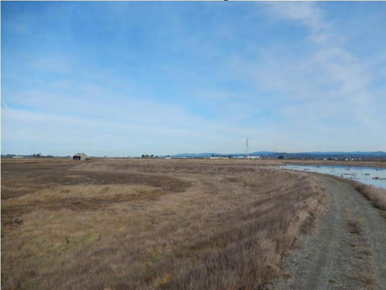
Site 9: CDFW western levee completed at 9' elevation and rocked – Dec. 2013 – North view
