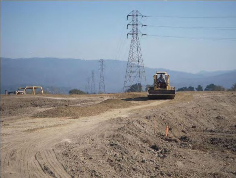
Site 6: Surfacing CDFW northern ecolevee – Oct. 2009 – East view
