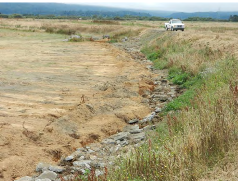
Site 17.1: City flood levee toe re-enforcement –Aug. 2013- Southeast view
