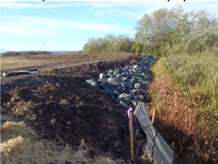
Site 17: Completed City flood levee rip rap installation –Aug. 2012 –Southwest view
