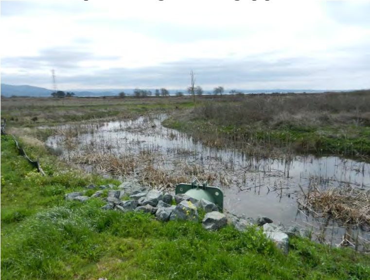
Site 18: Tide gate/drainage pipe installed in 2012 - March 2013 - South view
