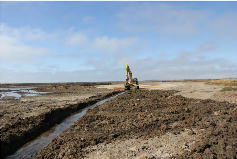
Site 11.1: Digging CDFW brackish pond input channel from slough –Oct. 2012 – Northwest view
