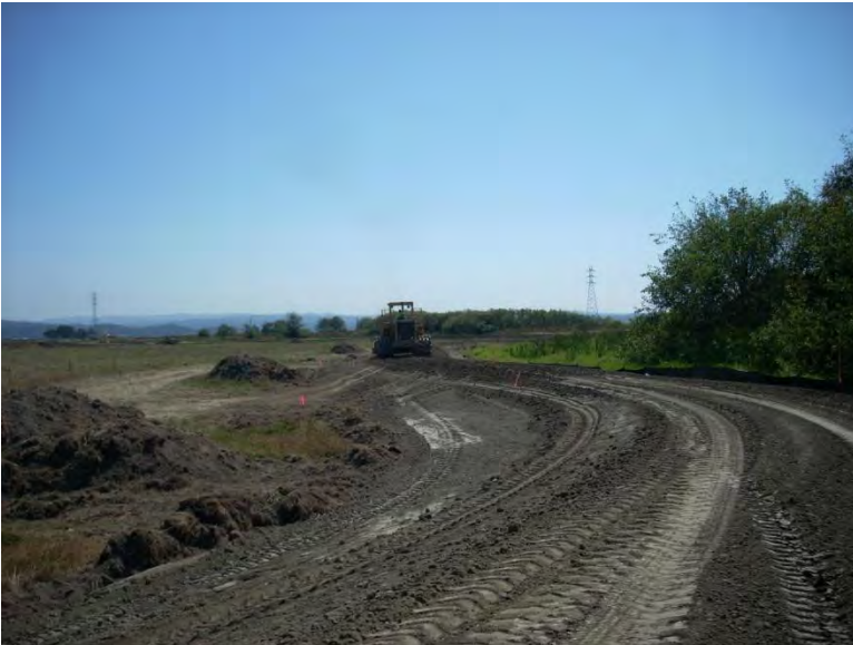
Site 17: Sheepsfoot compacting surface of City flood levee –Aug. 2012 –Southwest view
