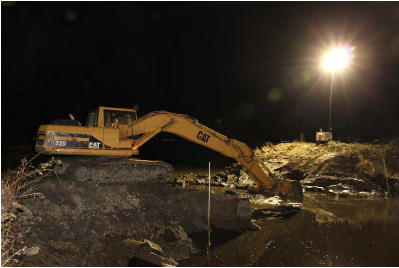
Site 19: Breaching McDaniel Slough and Humboldt Bay levee -Sept. 2013- Southwest view
