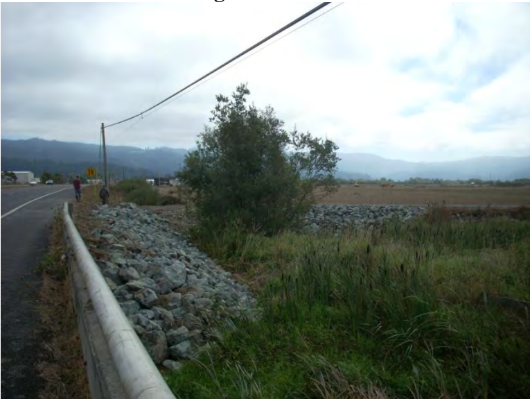
Site 16: Completed Hwy 255 and flood levee tie in with rip rap installation. One week before levee breach. –Sept. 2013 – East view
