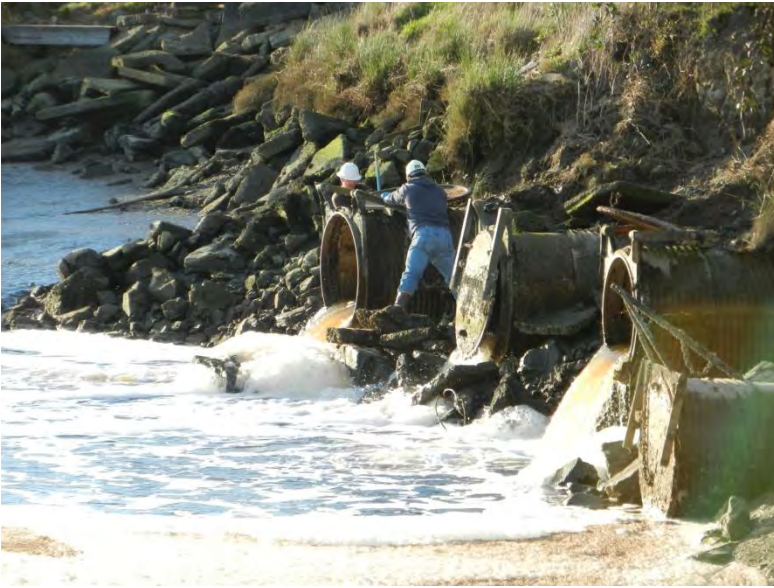
Site 19: Two of McDaniel Slough tides gates being chained open –Dec 2012 –West view
