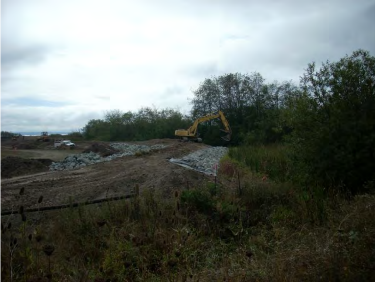
Site 17: City flood levee construction and rip rap installation – Aug. 2012 –Southwest view
