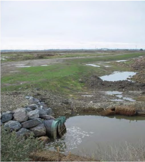
Site 13: Tide gate & slough crossing installed connecting CDFW flood levee to bay front levee – Nov. 2010 – North view
