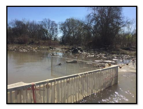
Close-up view of temporary fish barrier deployed at the fishway on the east section of Fremont Weir. The barrier is constructed of specially designed crowder racks and ¼ inch mesh beach seine. Photograph taken 14 March 2017.
