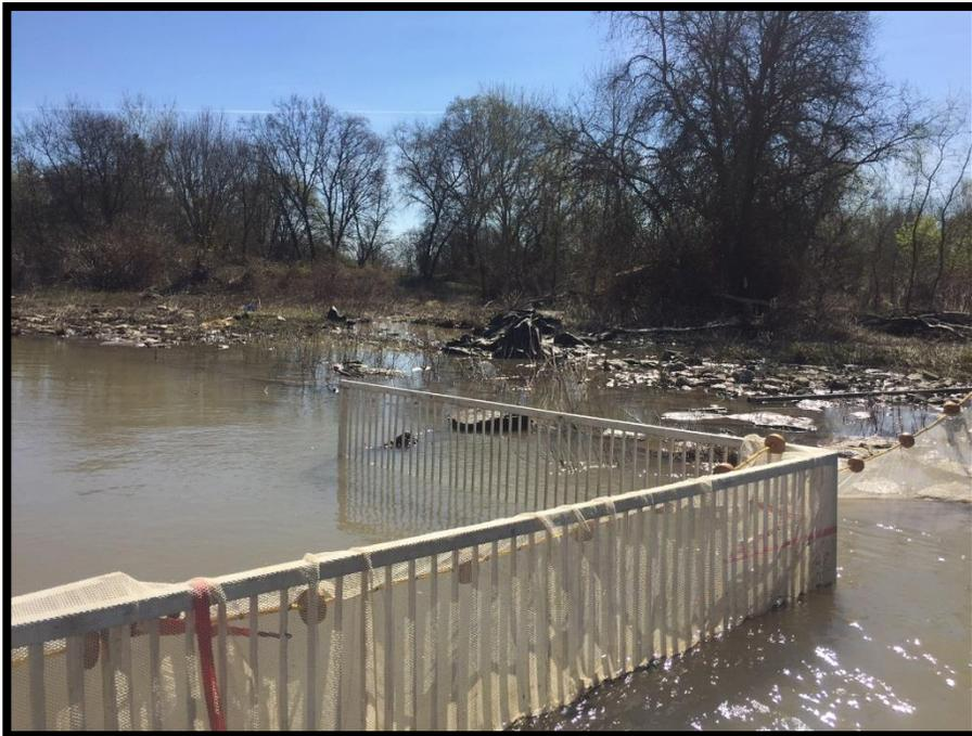
Close-up view of temporary fish barrier deployed at the fishway on the east section of Fremont Weir. The barrier is constructed of specially designed crowder racks and ¼ inch mesh beach seine. Photograph taken 14 March 2017.
