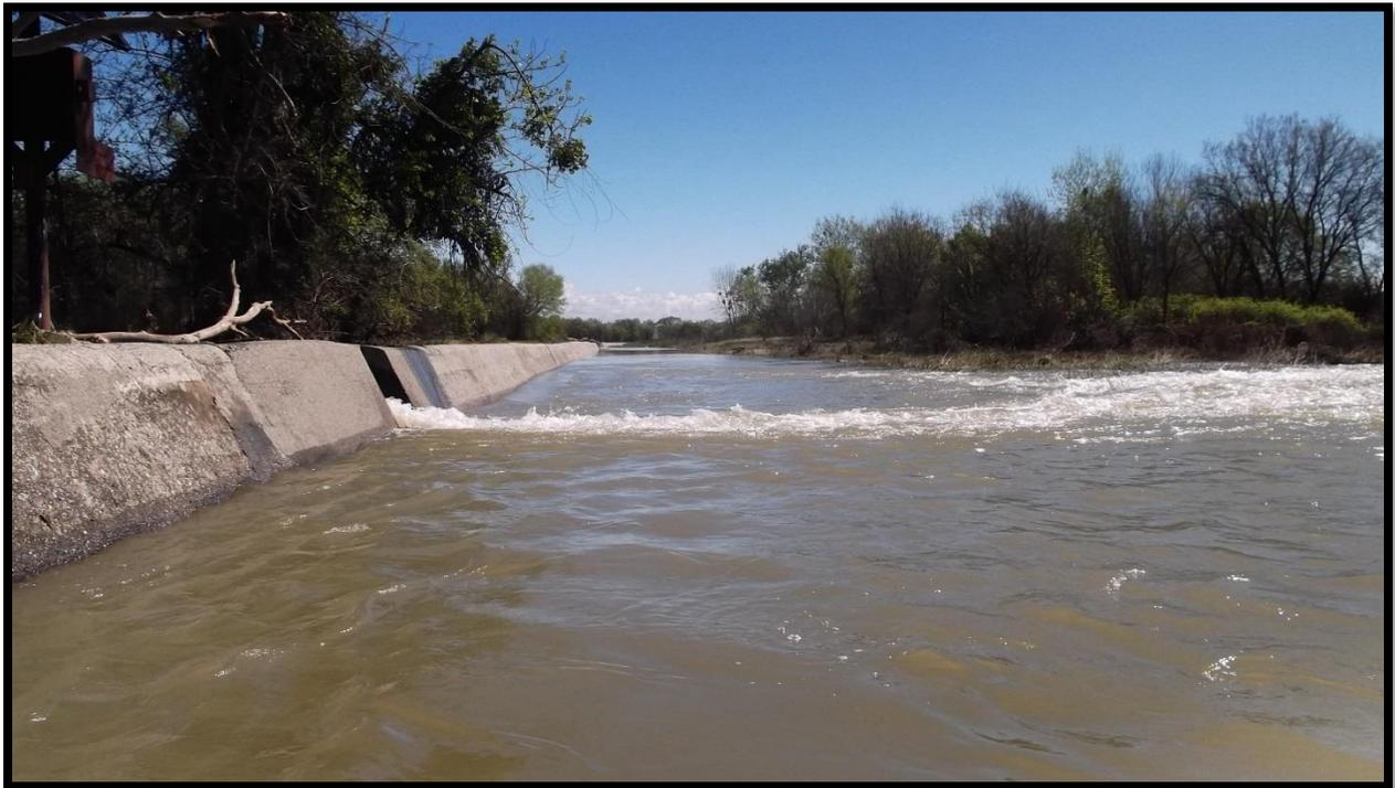
**Figure 3.** View of Fremont Weir during after cessation of overtopping event in March 2017. Flashboards have been removed to facilitate volitional fish passage to the Sacramento River prior to rescue operations.
