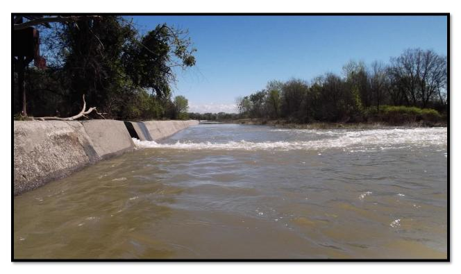
**Figure 3.** View of Fremont Weir during after cessation of overtopping event in March 2017. Flashboards have been removed to facilitate volitional fish passage to the Sacramento River prior to rescue operations.
