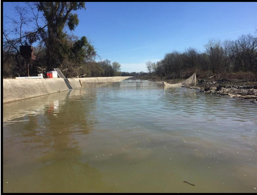
View of temporary fish barrier deployed at the fishway on the east section of Fremont Weir. Photograph taken 14 March 2017.
