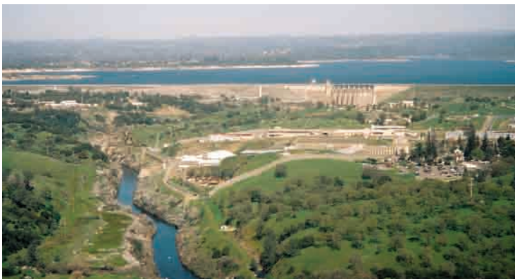
Folsom Dam looking eastward.
