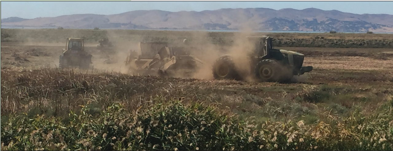
Low pressure grade tractors, cats, dozers, and scrapers laying the groundwork for restoring tidal action to the Tule Red property in Suisun Marsh. Photo: Westervelt Ecological Service
