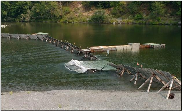
Figure 4. Willow Creek weir in 2018. Note the floating boat gate and tunnel with camera box downstream of trap.
