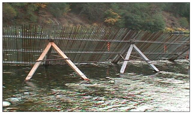
Figure 2. Photograph of Alaskan-style weir, tripods, support channels, and conduit (looking upstream).
