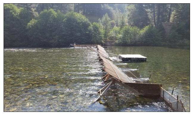
Figure 3. Junction City weir (JCW) configuration in 2018 after the JW 30 rebuild. This shows the weir in trapping mode. Stream flow is right to left.
