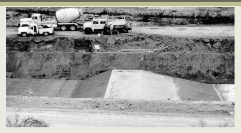
A broad crested weir (BCW) being built. We will be installing BCW's to increase the accuracy of measuring how much water 3 state wildlife areas are receiving.
