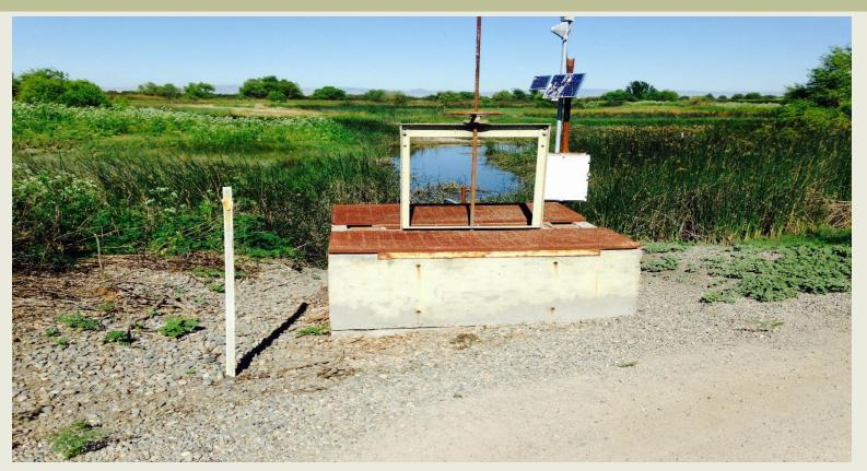
The current drainage structure at Buttonwillow Lakes Dam on Los Banos Wildlife Area. We will rebuild the dam to allow for a dropdown gate to be installed.
