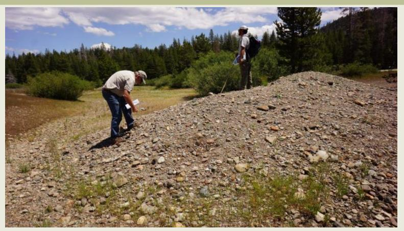
Gravel push-up dam in the historic channel of Lacey Creek through Upper Lacey Meadow, used to divert the stream into the present day unstable channel.
