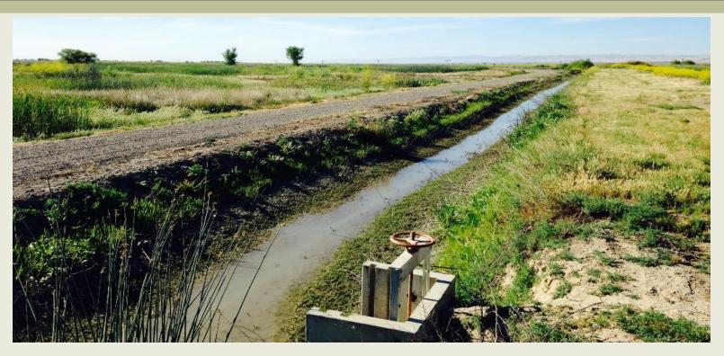
A section of the main delivery ditch bank on the Gadwell Unit will be built up to allow the wildlife area staff to build up head pressure to push water into adjacent units. Currently, water almost floods over the existing ditch bank (left side of picture) when building up head pressure.
