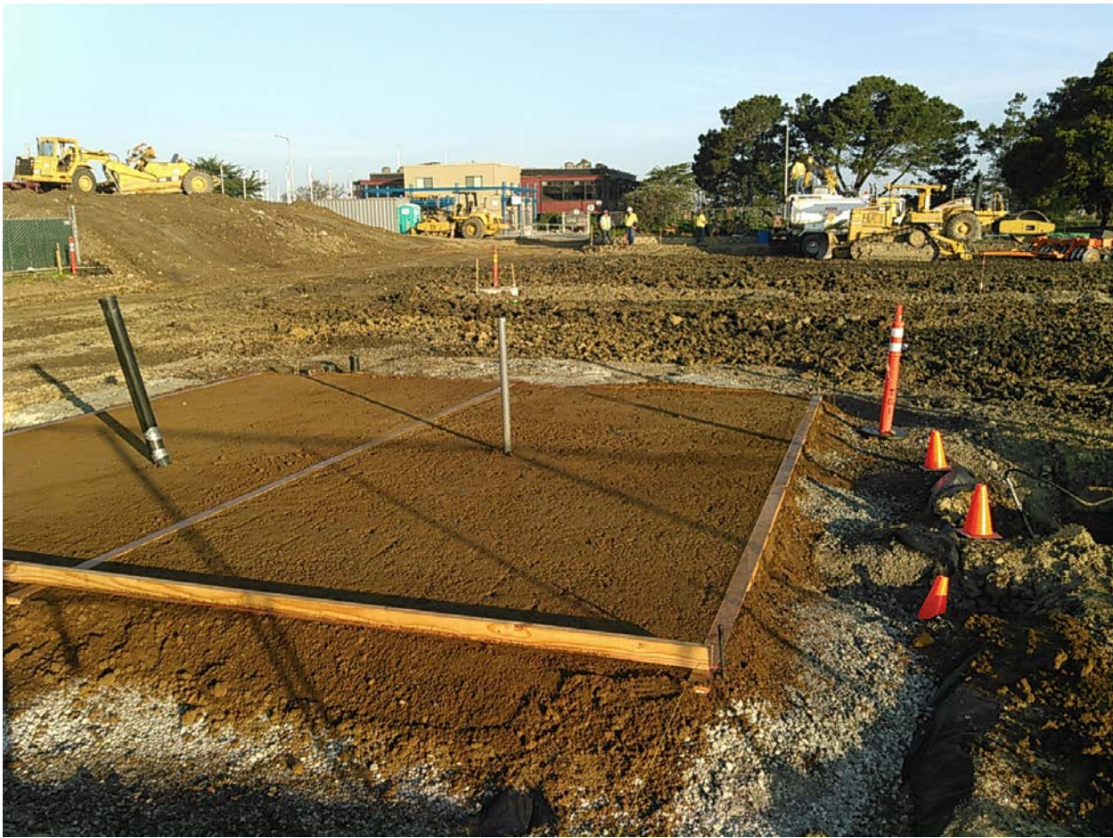
Image 4: South Cove East Parking Lot – Complete final base layer for new restroom (Photo by D. Sheils).
