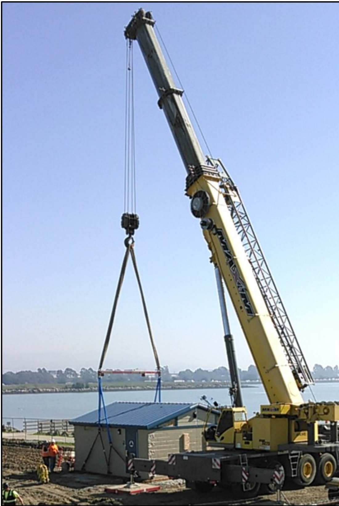
Image 6: South Cove East Parking Lot – Installing the new pre-fabricated public restroom by crane at the site (Photo by D. Sheils).
