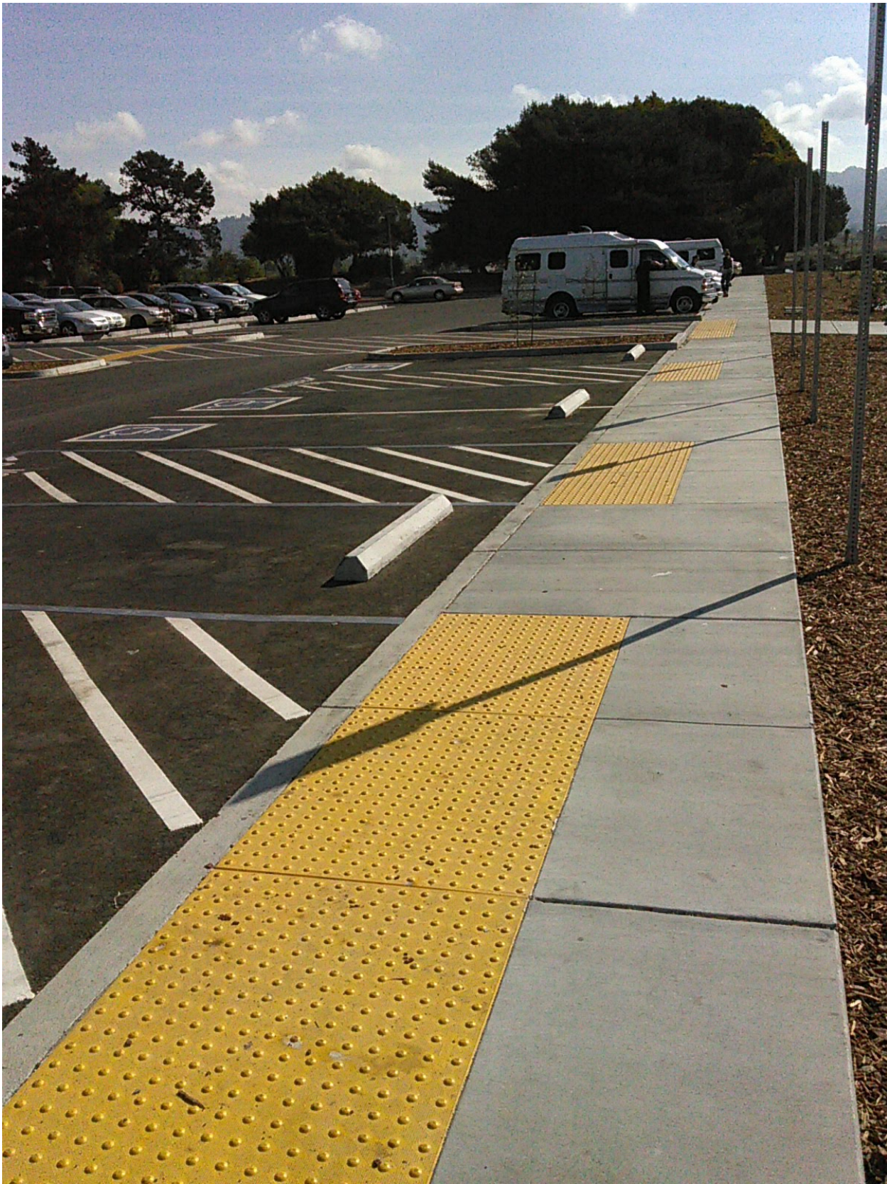
Image 12: South Cove East Parking Lot – The fully asphalted and striped accessible path of travel from the ADA parking slots to the new public restroom (Photo by D. Sheils).
