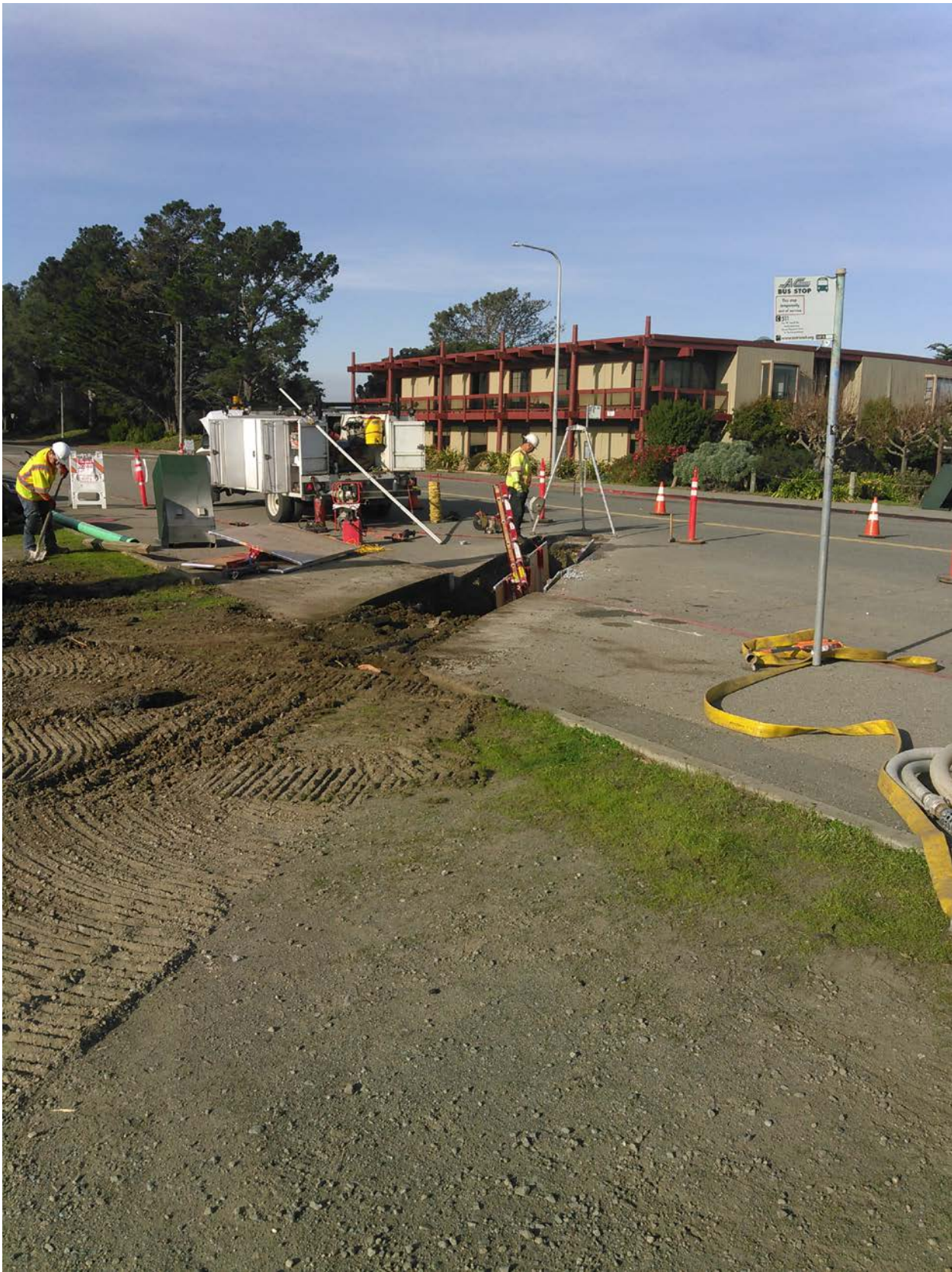
Image 1: South Cove East Parking Lot – Excavating the new sanitary sewer line for the new public restroom, starting at the mainline manhole at University Ave, 10 feet below grade (Photo by D. Sheils).
