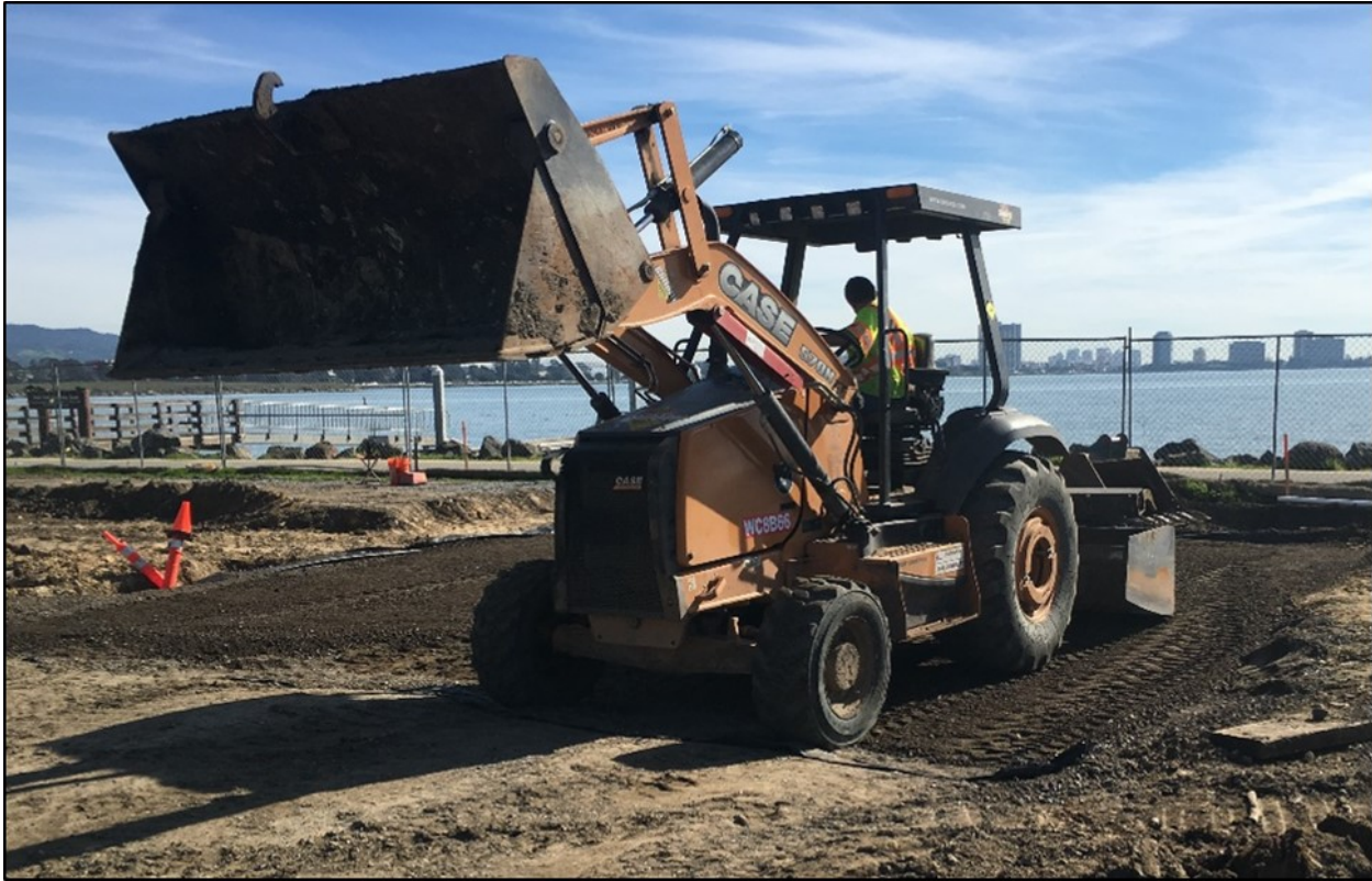
Image 3: South Cove East Parking Lot – Compacting and stabilizing existing subsoils atop Bay muds (Photo by D. Sheils).
