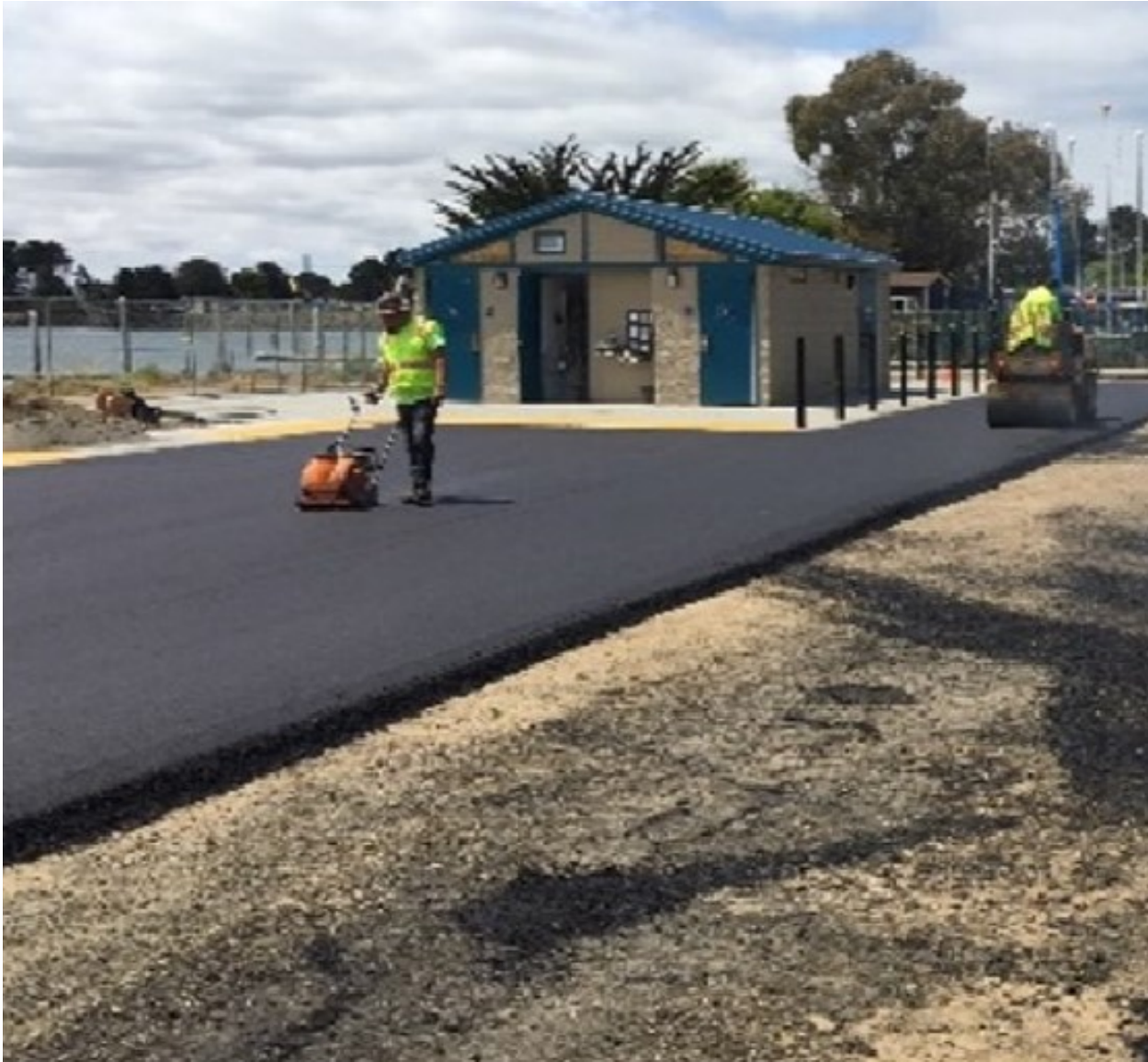
Image 11: South Cove East Parking Lot – New asphalt paving atop the stabilized base layer to provide ADA accessible parking slots adjacent to the new public restroom (Photo by D. Sheils).
