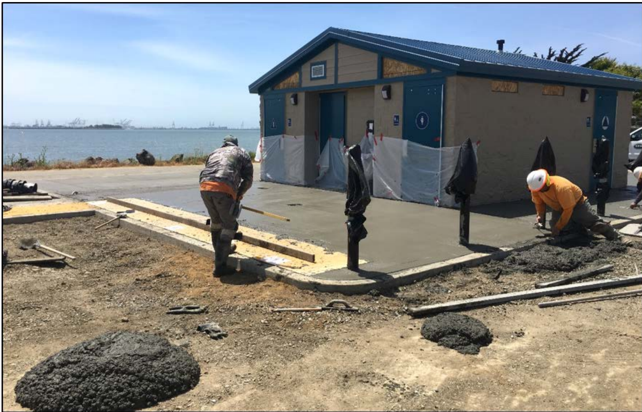
Image 9: South Cove East Parking Lot – Installing the new concrete restroom plaza adjacent to the new ADA accessible parking slots with accessible path of travel to the new public restroom (Photo by D. Sheils).
