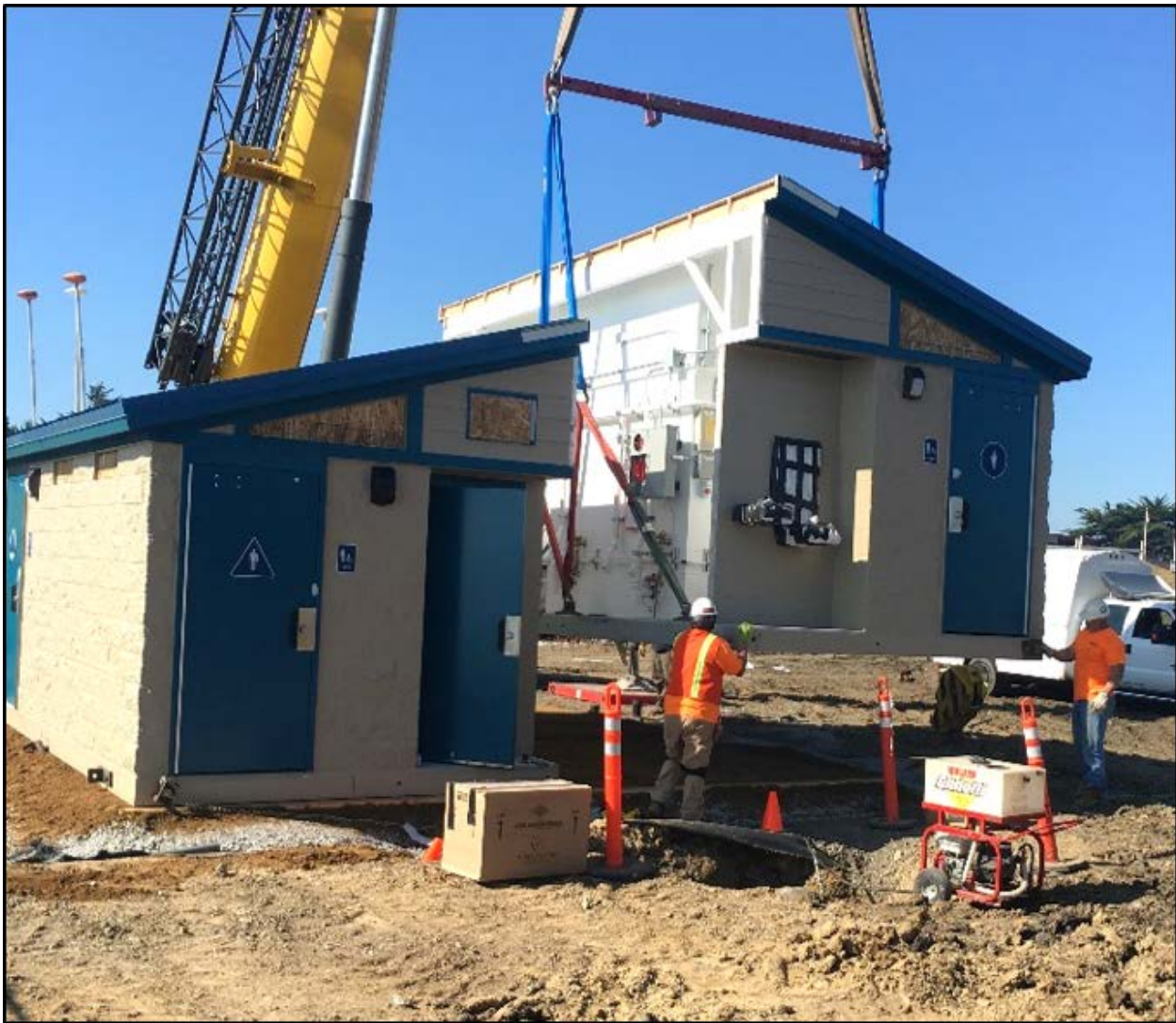
Image 5: South Cove East Parking Lot – Installing the new pre-fabricated restroom by crane at the site. The restroom building is constructed in two sections in order to meet highway transportation requirements (Photo by D. Sheils).
