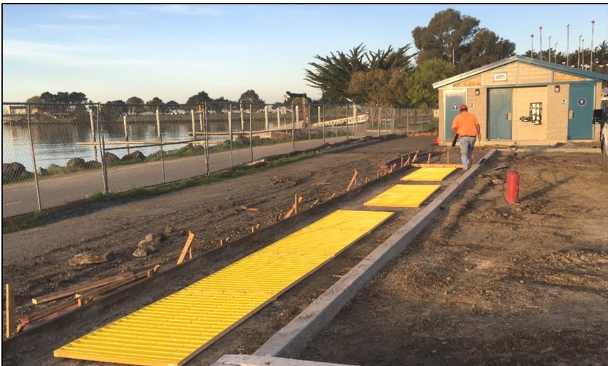
Image 10: South Cove East Parking Lot – Installing truncated dome detectable surfaces for the new accessible concrete sidewalk path of travel to the new public restroom (Photo by D. Sheils).
