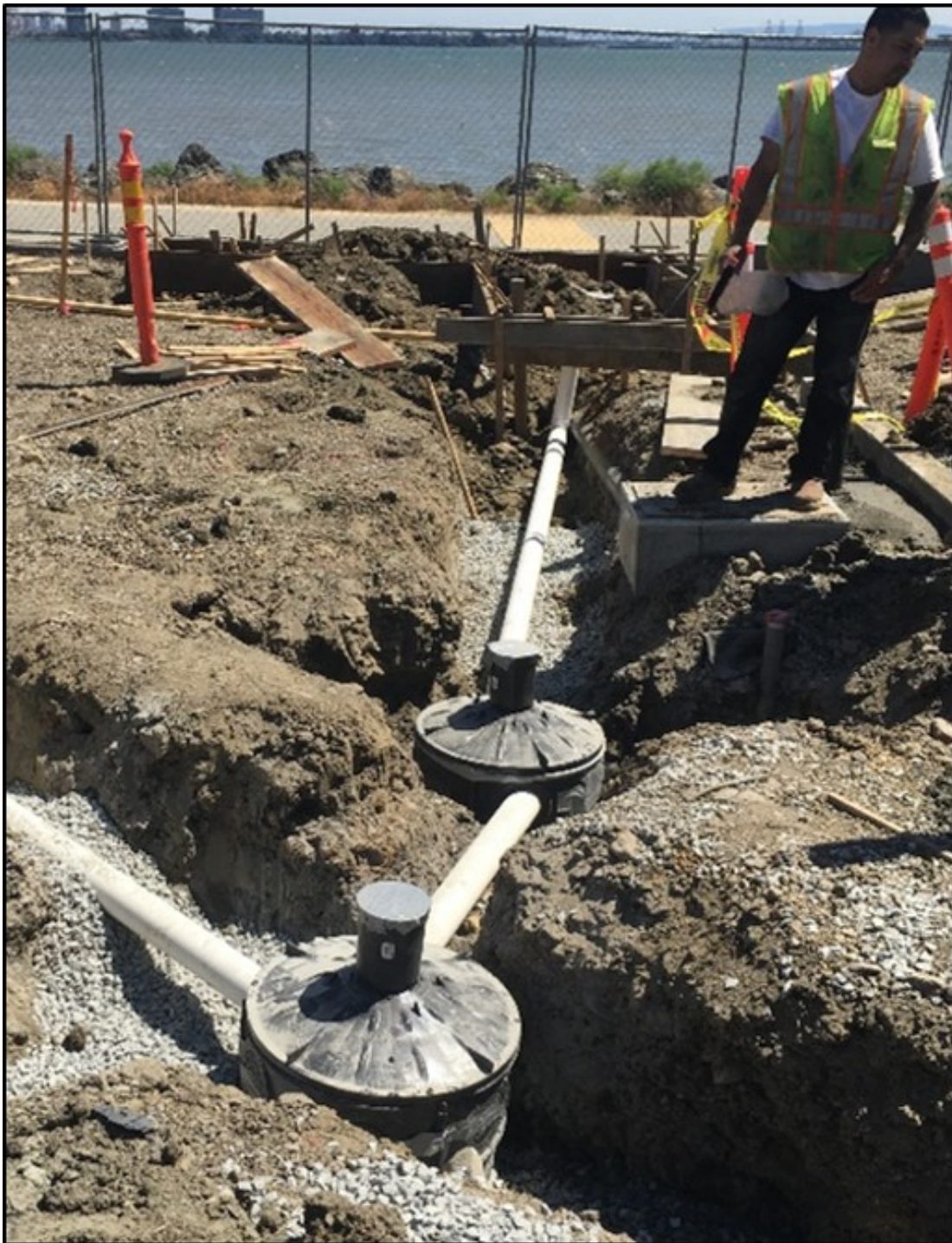
Image 8: South Cove East Parking Lot – Installing the drainage system for the new concrete restroom plaza area and outdoor washdown area at the restroom (Photo by R. Miller).
