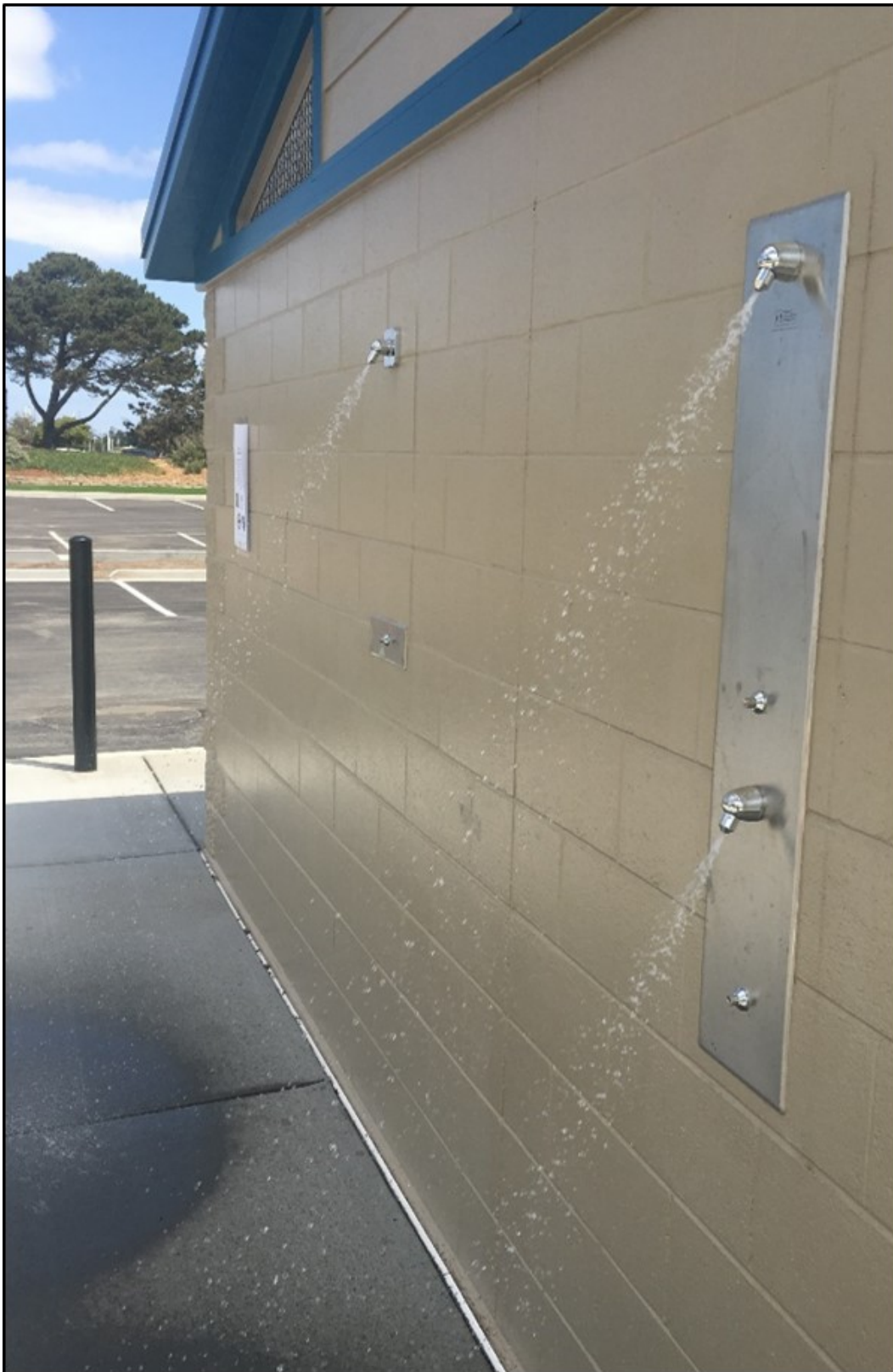
Image 14: South Cove East Parking Lot – Post renovation, there is a new outdoor washdown at the new public restroom with time-limited pushbuttons for water savings. There is also an ADA accessible pushbutton (Photo by D. Sheils).
