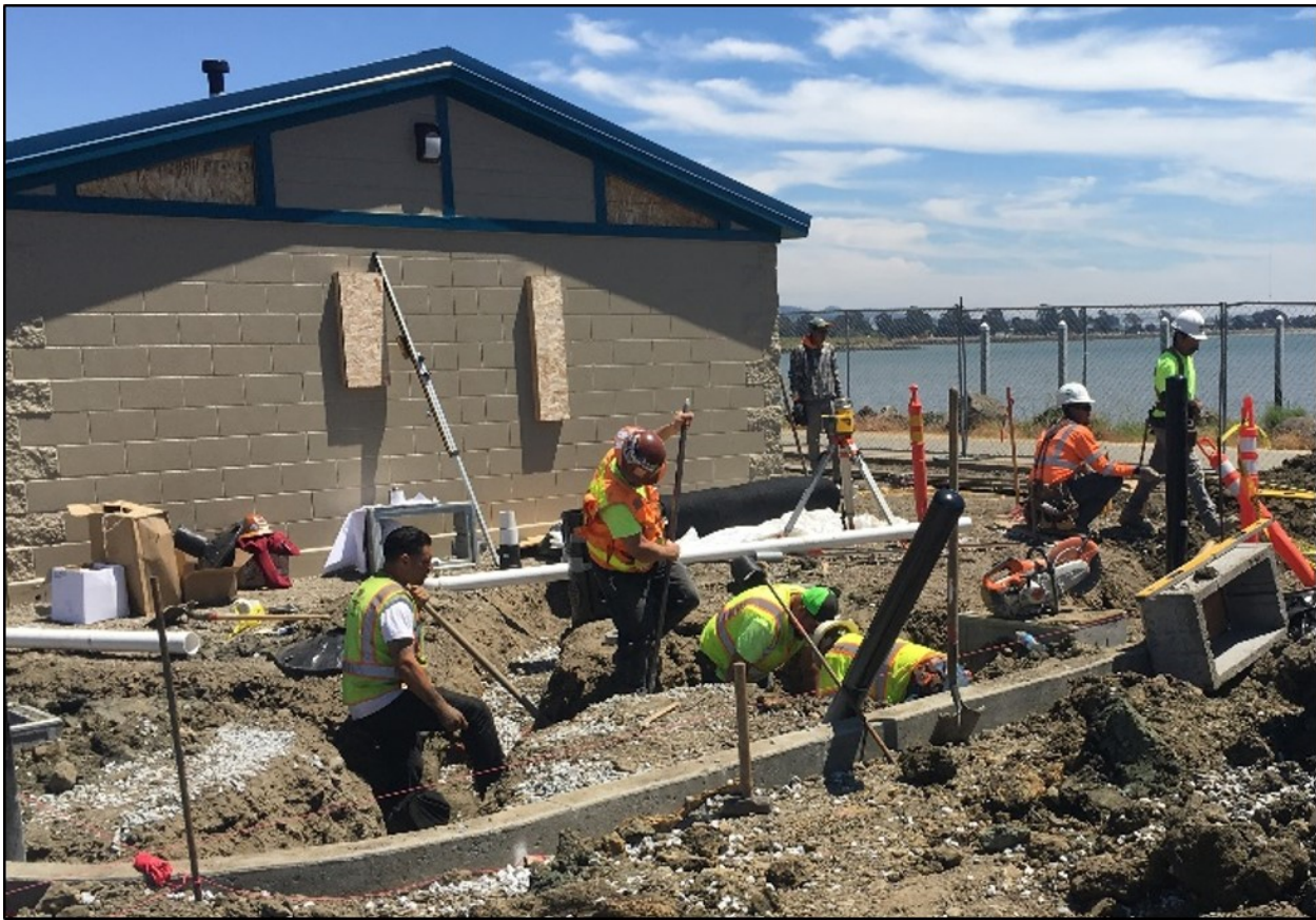
Image 7: South Cove East Parking Lot – Installing the drainage system for the new concrete restroom plaza area and outdoor washdown area at the restroom (Photo by R. Miller).
