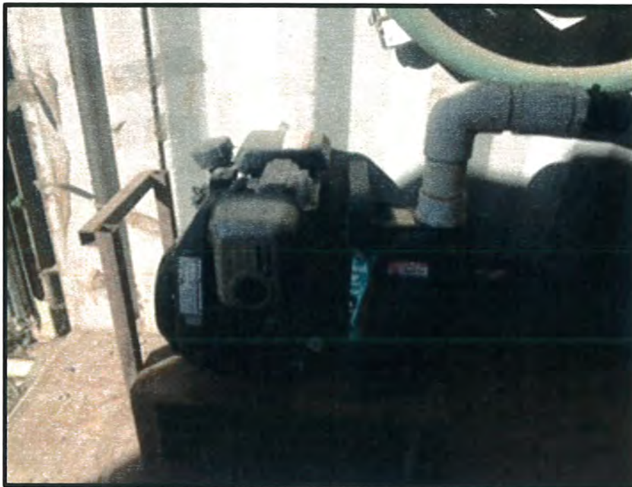
Figure 23. Pump used to Operate the Clam Rake
