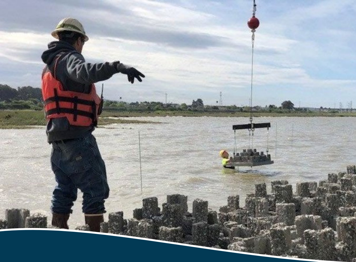
Workers with contractor Triton Marine lower one of 350 oyster reef structures into the water near Giant Marsh to create a “living shoreline” supporting local fish and wildlife. Photo by California Coastal Conservancy
