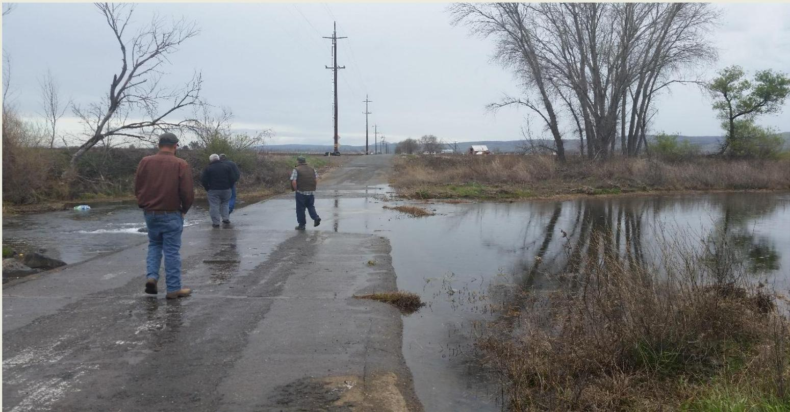
Dye Creek running over Shasta Boulevard after a winter storm event. The current culverts are insufficient to handle the average amount of water flow.
