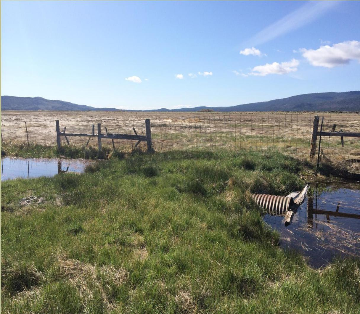
Failing corrugated metal pipe culverts, set at incorrect elevations will be replaced with HDPE pipe
