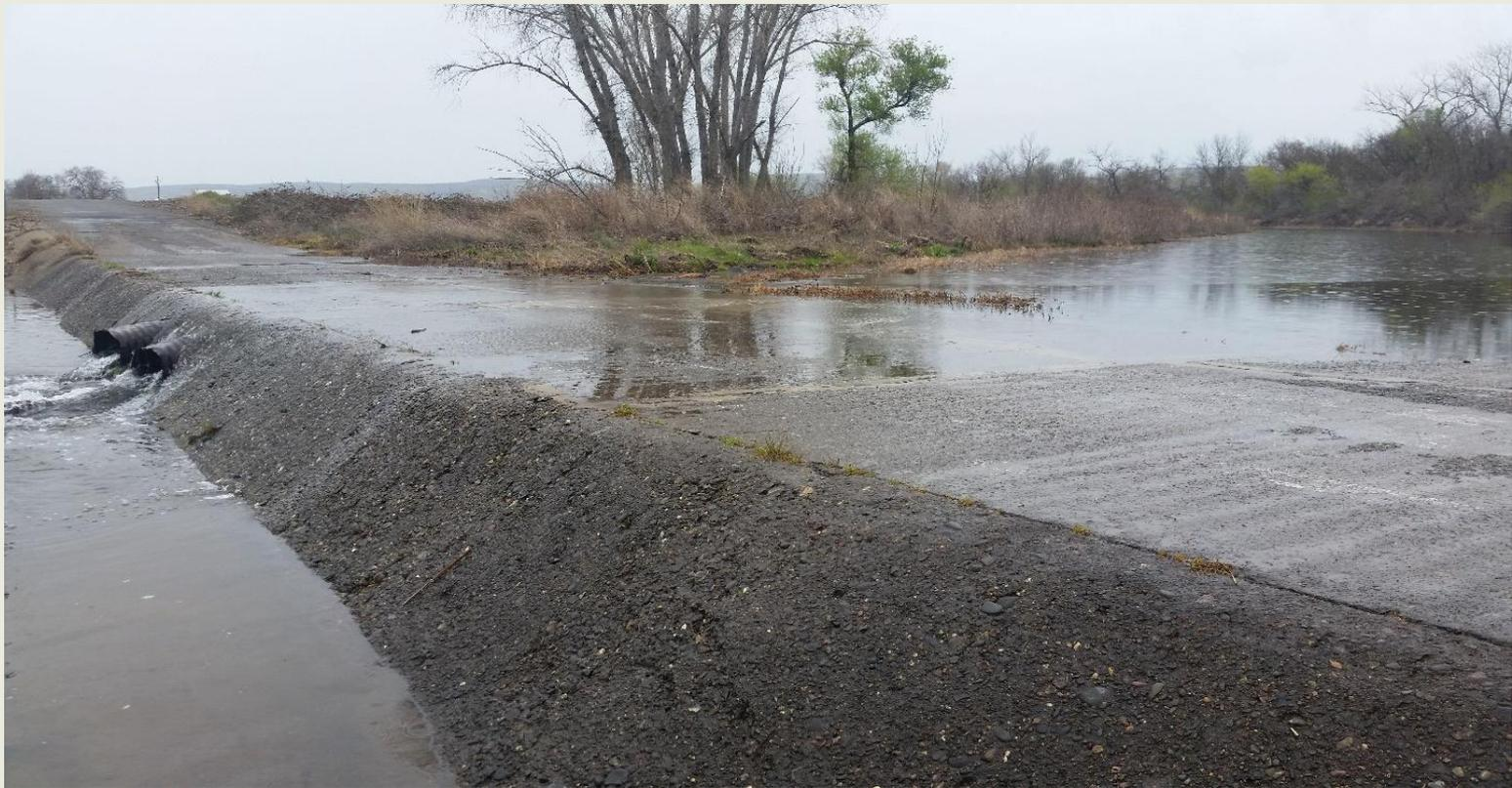
The current low water crossing with its undersized 12-inch diameter culverts has filled with sediment and is impeding fish passage.
