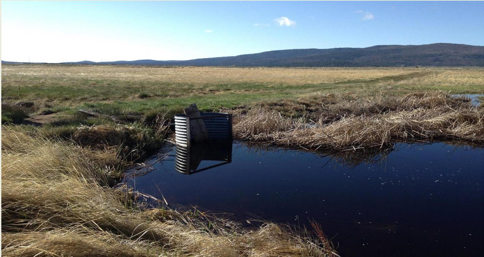
Old corrugated metal half-round risers will be replaced with new cast concrete weirs
