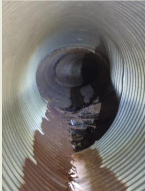
Photo 2: Interior of culvert showing damage to corrugated metal pipe
