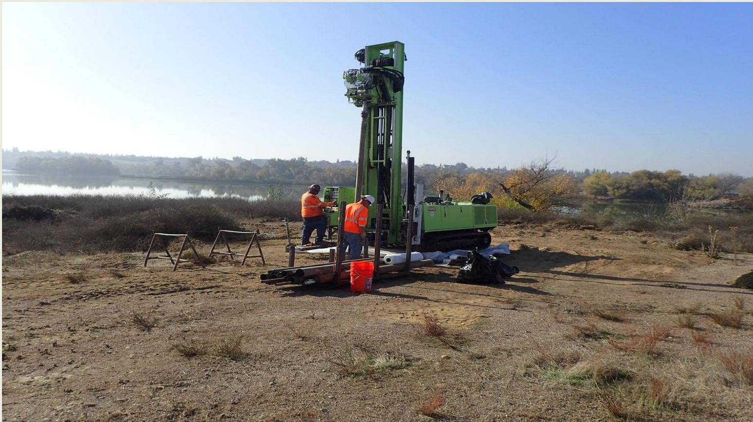
Pond berm drilling and substrate sampling in 2017 during preliminary study phase
