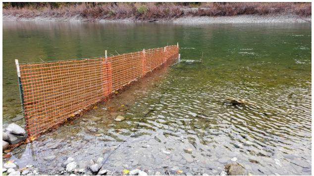
5.) 12.01.2019. Panels with buildup that must be removed early during season. As flows increase, detritus gets flushed downstream and eventually stops collecting on panels.
