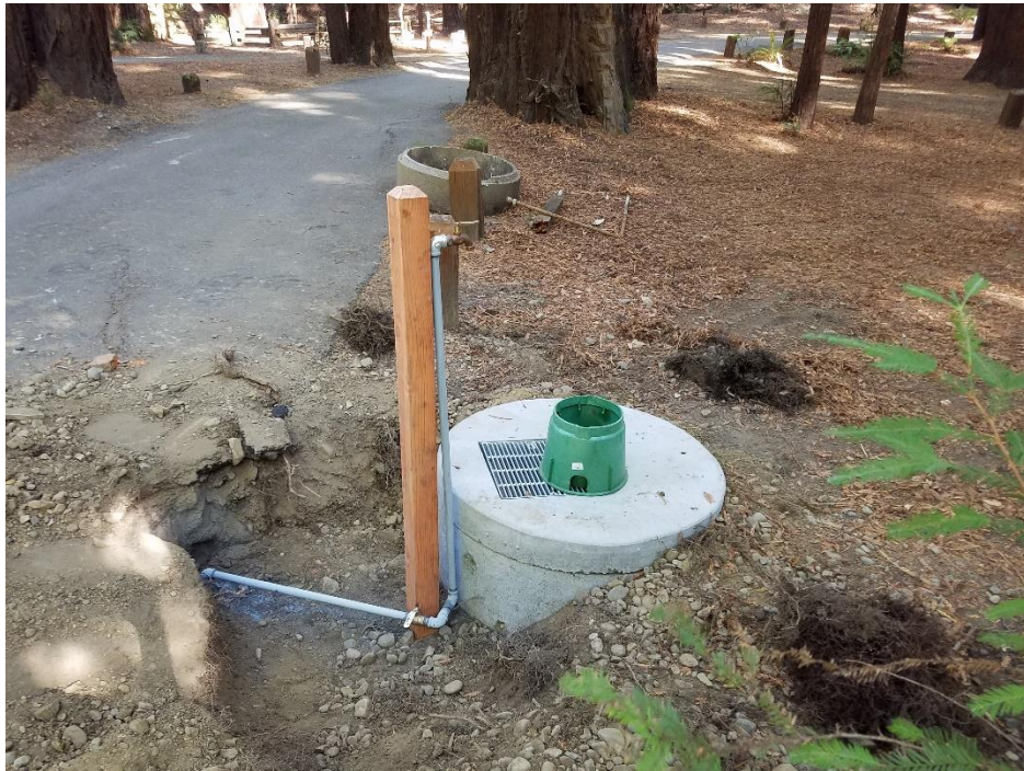
Photo 18. New grated drain at Burlington Campground in October 2017.
