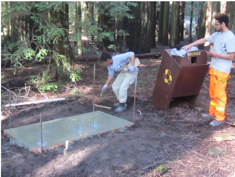
Photo 6. AmeriCorps crew installing concrete pads at Marin Group Camp.
