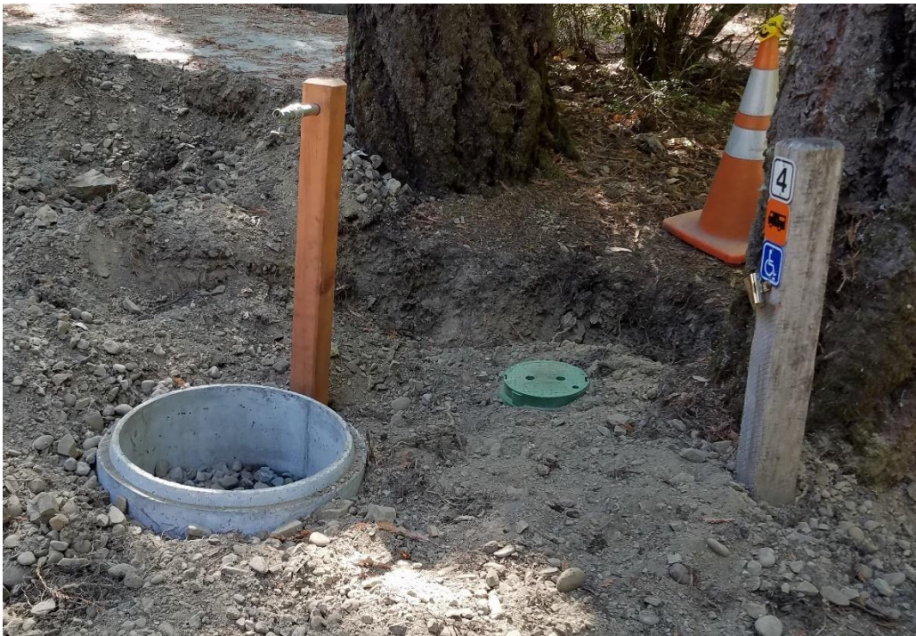
Photo 30. New grated drain installation at Hidden Springs Campground in 2018
