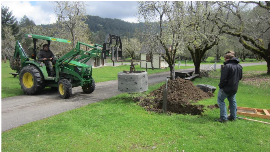
Photo 12. State Parks staff replacing drain casings at Cuneo Horse Camp.
