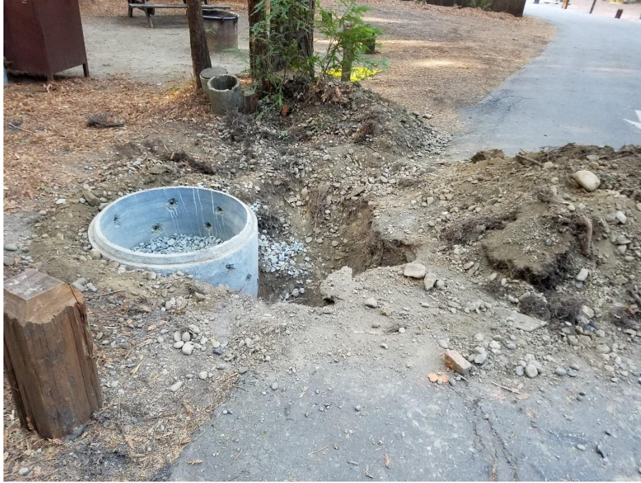
Photo 17. Installation of new grated drain casing at Burlington Campground in October 2017.
