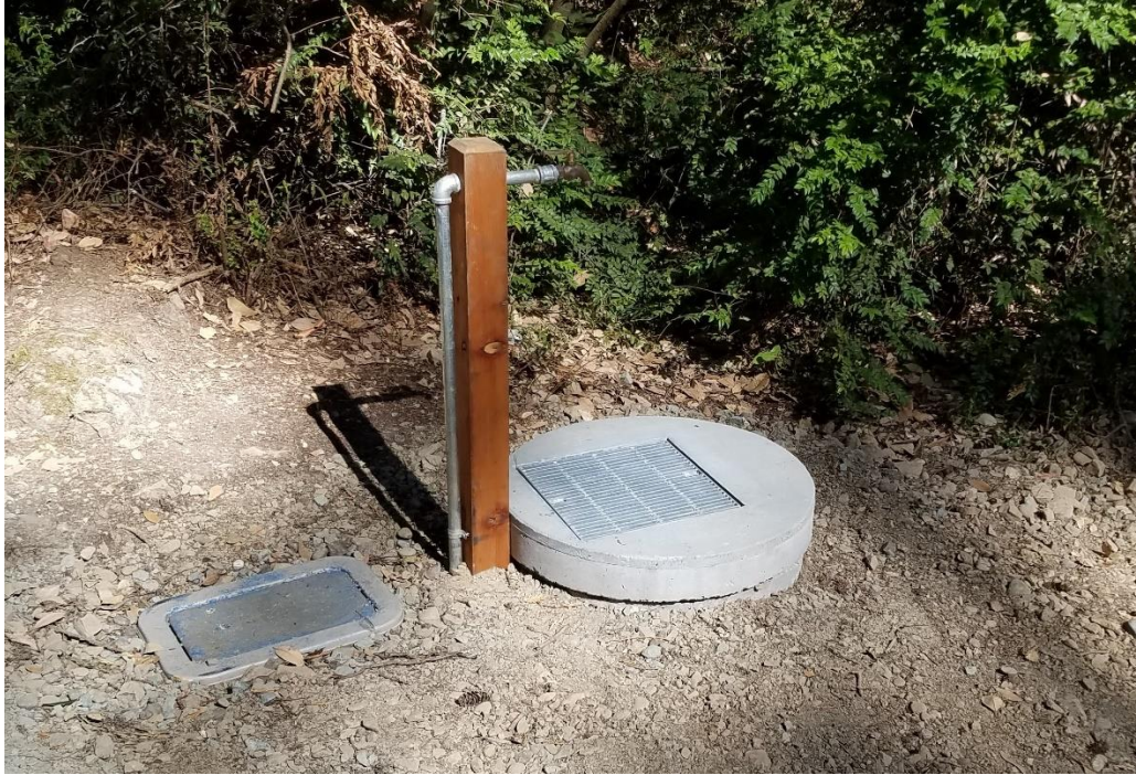
Photo 31. New grated drain at Hidden Springs Campground in 2018.
