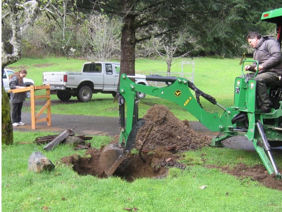
Photo 13. State Parks work crew installing new drain casings at Cuneo Horse Camp.
