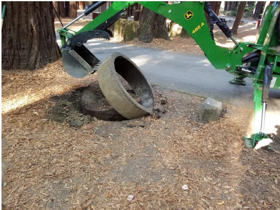
Photo 16. Excavation of old French drain at Burlington Campground in October 2017.
