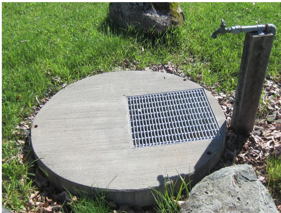
Photo 1. New wildlife-proof grated water drains at Cuneo Horse Camp.
