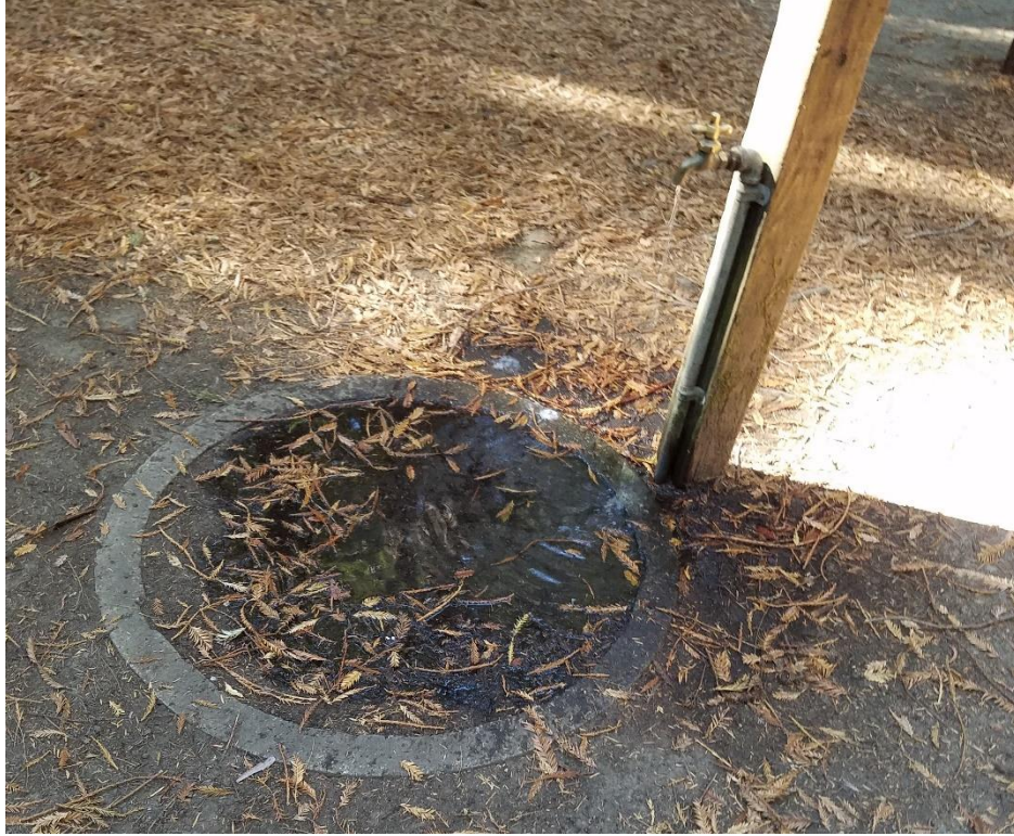
Photo 15. Old French drain at Burlington Campground in October 2017.
