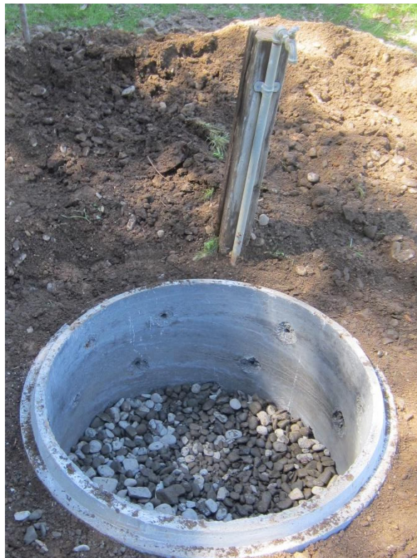
Photo 14. New drain casing at Cuneo Horse Camp (without grated lid on).
