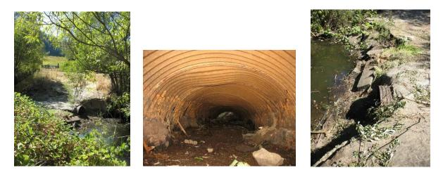
Photos (L to R): BEFORE -- Collapsed ford and culvert from right bank of Green Valley Creek; Culvert interior; Crossing and culvert from left bank
