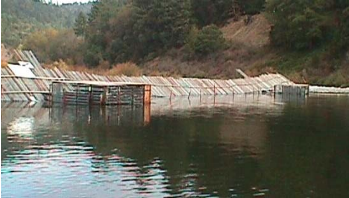
Figure 4. Photograph of Alaskan weir showing the trapping boxes on the upstream side of the weir.
