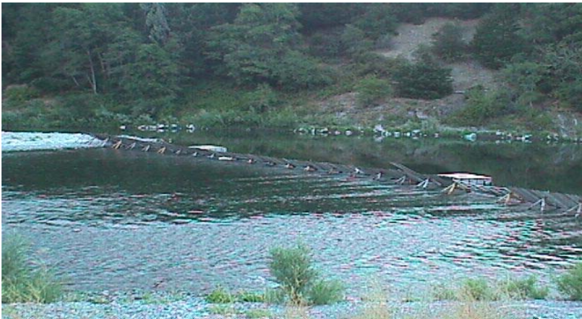
Figure 3. Photograph (taken downstream) of Alaskan weir. Note the boat gate (right side of picture).
