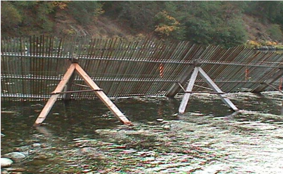
Figure 2. Photograph of Alaskan style weir tripods, support channels and conduit.
