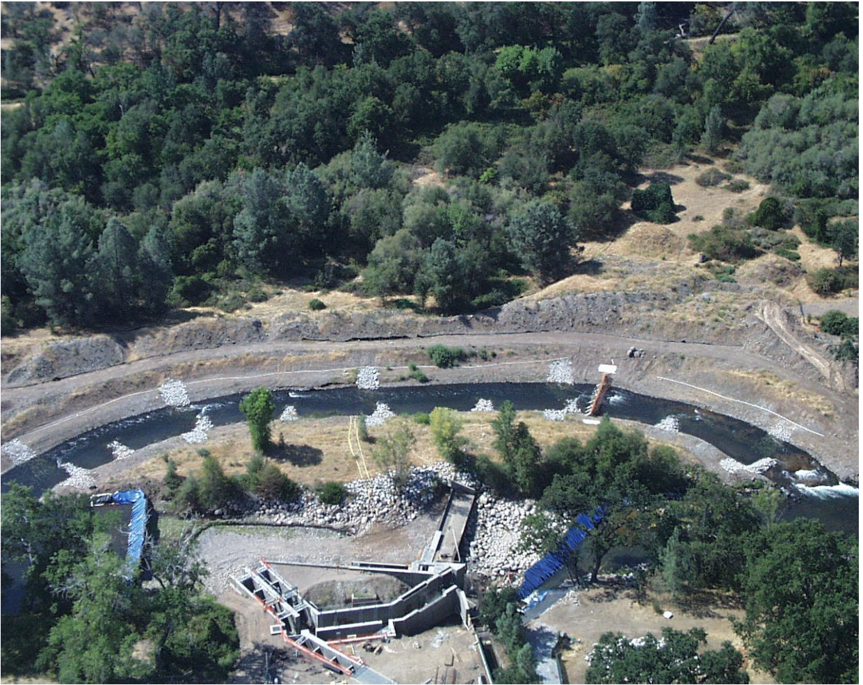
Appendix Figure E9. Aerial view of construction of new fish ladder at CNFH in 2008.
