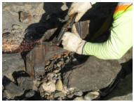
**Figure 1: Cutting Low Flow Notch**
