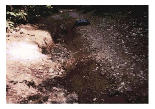
Figure 21. During heavy rainfall, soil from this 1 ft deep gully on a mining access road goes directly into Briggs Creek. Gully is actively headcutting uphill on 20 percent grade.
