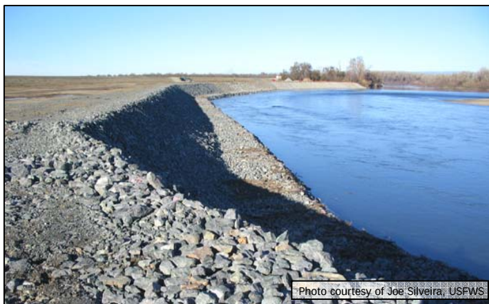
Channelization and bank revetment
