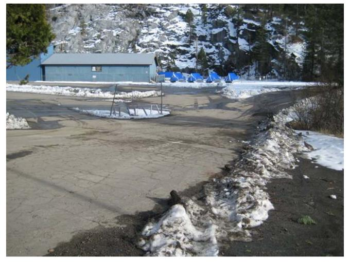
Broken asphalt to be repaired and the storm drain to be replaced (in center of picture)
