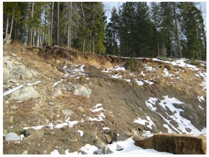
• Failed slope to be repaired in upper parking lot area
