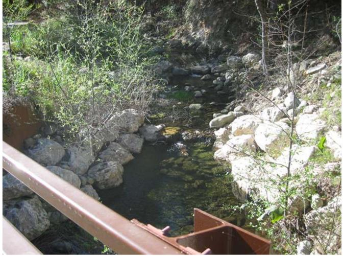
Looking upstream at crossing #6. Note grade control structures creating step pools for steelhead
