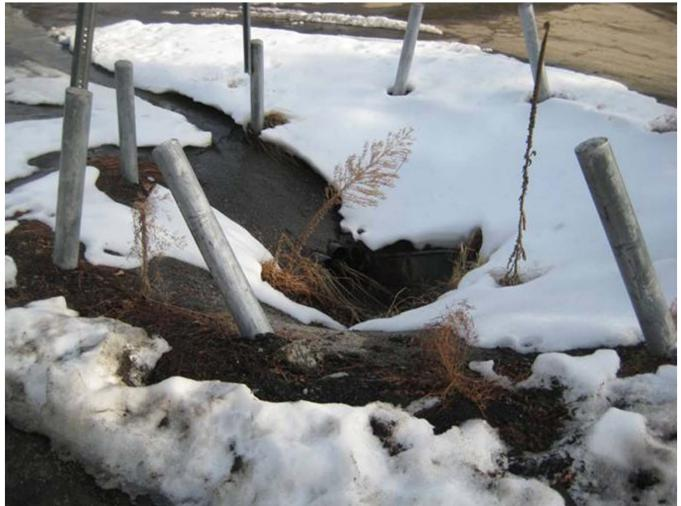
Storm drain to be replaced with integrated oil/sand separator drain
