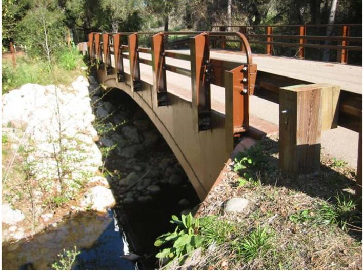
Bottomless arched culvert constructed in 2008 at crossing #6
