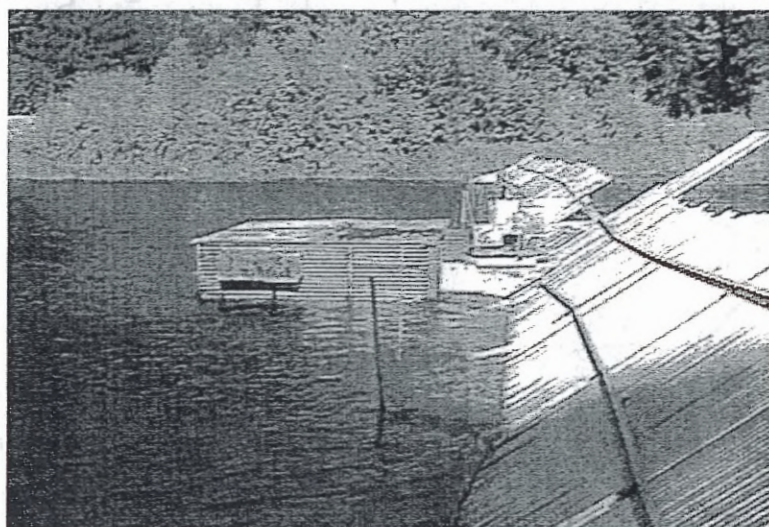
Figure 4. Photograph of Alaskan weir showing the trapping box on the upstream side of the weir.
