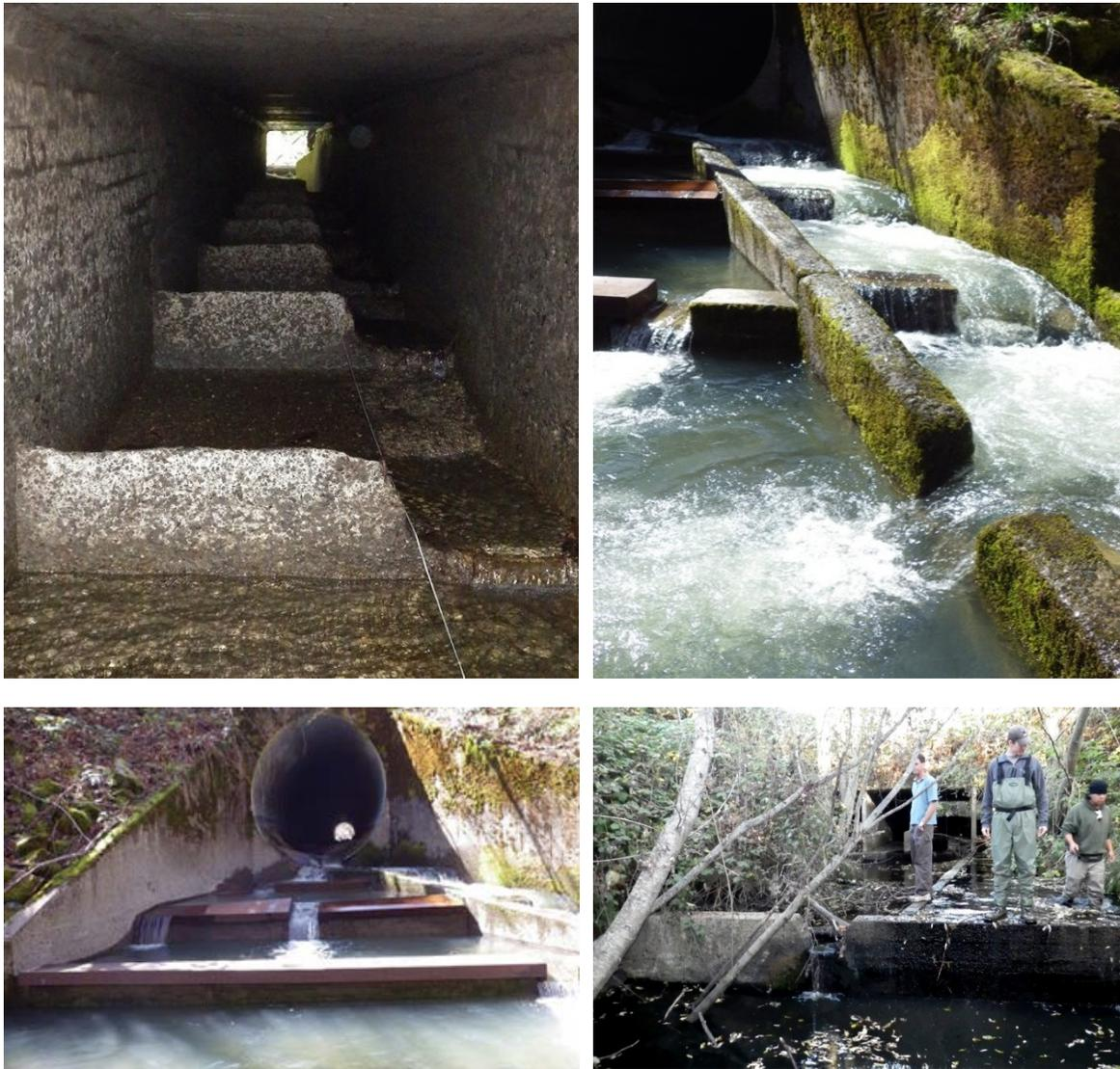
**Figure 2-5.** Examples of internal structures and modifications at road crossings in the Eel River basin. Internal baffles (top left; Fish Creek, PAD 707157), step-pool fishways at outlet (top right and bottom left; Elk Creek, PAD 707107), and tailwater control weir (bottom right; Rohner Creek at 12<sup>th</sup> St. in Fortuna, CA).
