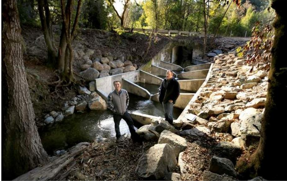
Figure 5-1. Example pool-weir fish ladder designed to improve salmon passage, but not well designed for Pacific lamprey passage. Source: <http://www.pressdemocrat.com/article/20140109/articles/140109595>
