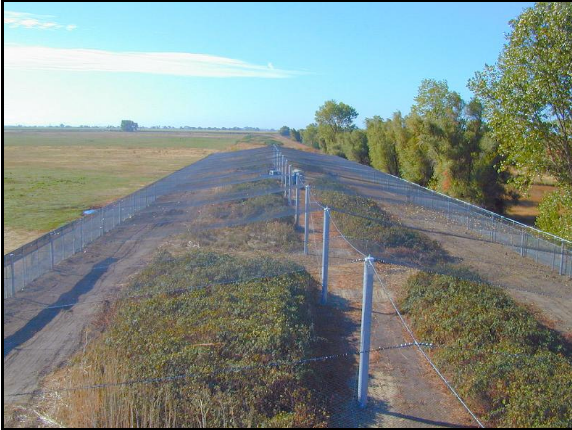
Figure 3. Photo of a portion of a pen for controlled propagation of riparian brush rabbits at Pond 6. The pen is approximately 530 feet long, 100 feet wide, and the side fencing is about 7 feet high. The top is covered with netting to prevent raptors from entering. Sides are topped with sheetmetal, shown on the left, but not yet installed on the right. For scale, two vehicles are parked near the center line (photo by L.P. Hamilton).
