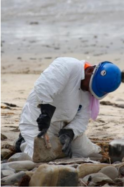
Beach uses a wire brush and other tools to scrape oil from cobble rock, Goleta, Calif., June 10, 2015. Environmental sensitivity of the site, heavy equipment cannot be used. Photo by Valerie Kushnerov, City of Goleta.
