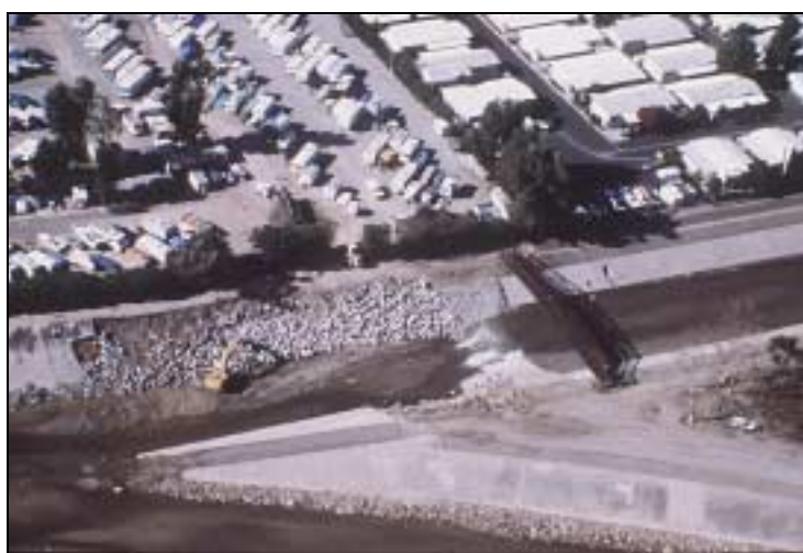
Photo 3. Downstream of San Juan Creek-Trabuco Creek confluence – post-1998 floods
