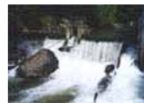
Photo 4-1 Battle Creek Salmon and Steelhead Restoration Project
