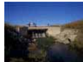
Photo 4-19 Lower Putah Creek—check dam (Yolo County)/Joe Krovoza photo
