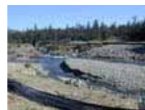
Photo 4-8 Clear Creek after removal of armored gravel berm /DWR photo
