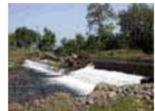
Photo 4-10 Mill Creek—Ward Dam (Tehama County)
