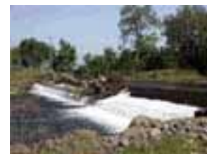
Photo 4-9 Deer Creek—Stanford-Vina Ranch Diversion Dam /Photo
