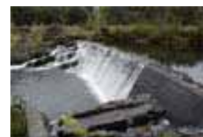
Photo 4-14 Cosumnes River—South Granlees Diversion Dam (Sacramento County)/DWR photo
