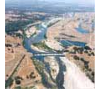
Photo 4-11 Yuba River— Daguerre Point Dam
