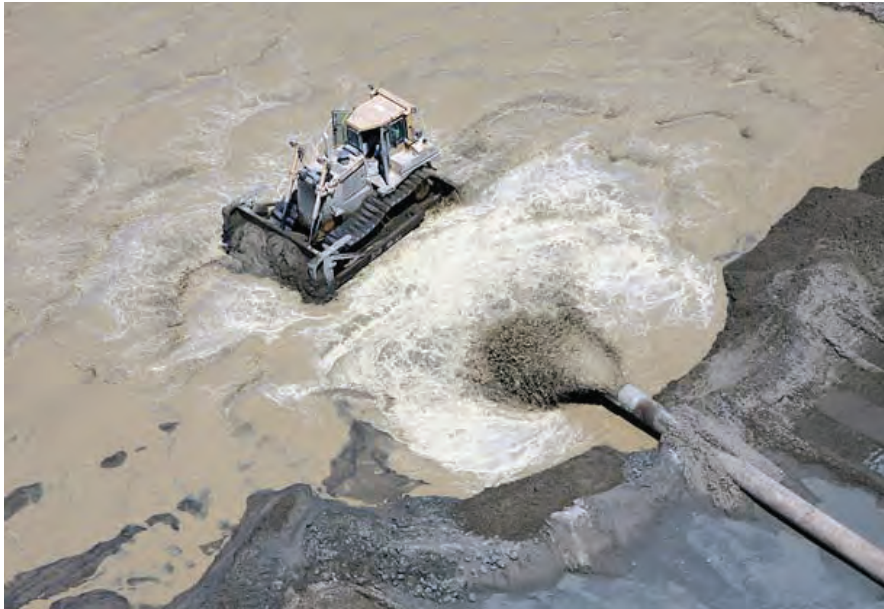
Photo A. Bulldozer clearing pipe discharge http://baynature.org/
