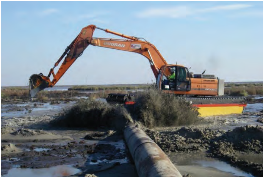
Photo C. Excavator clearing pipe discharge
