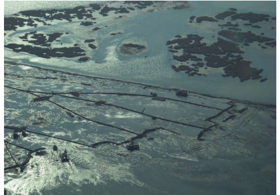
Photo B. Hydraulic placement
