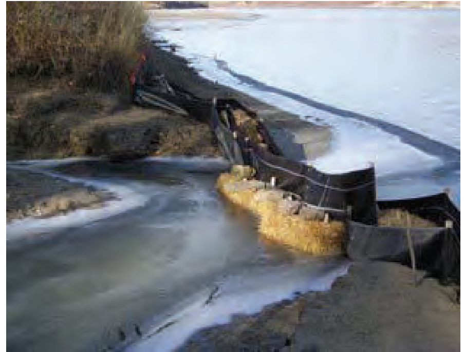
Photo B. Turbidity control with containment fencing
