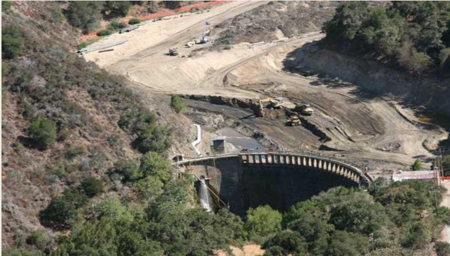
Sediment removal behind dam
