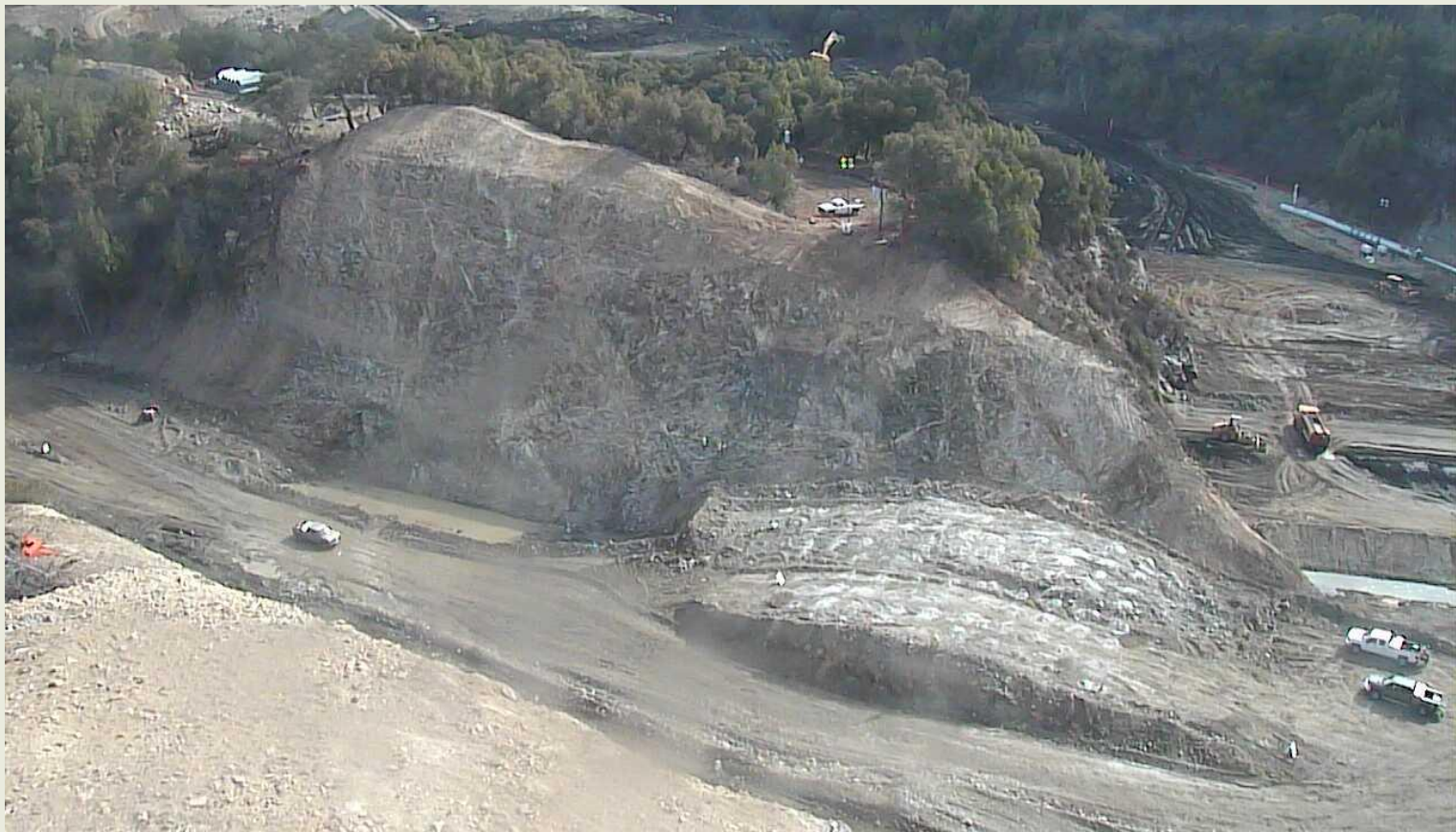
Reroute channel, October 2014
