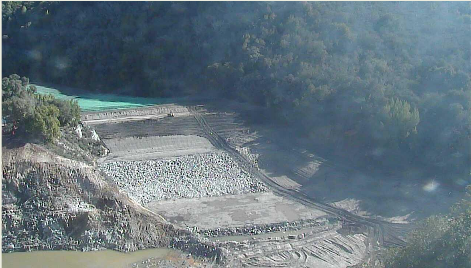
Diversion dike, December 2014
