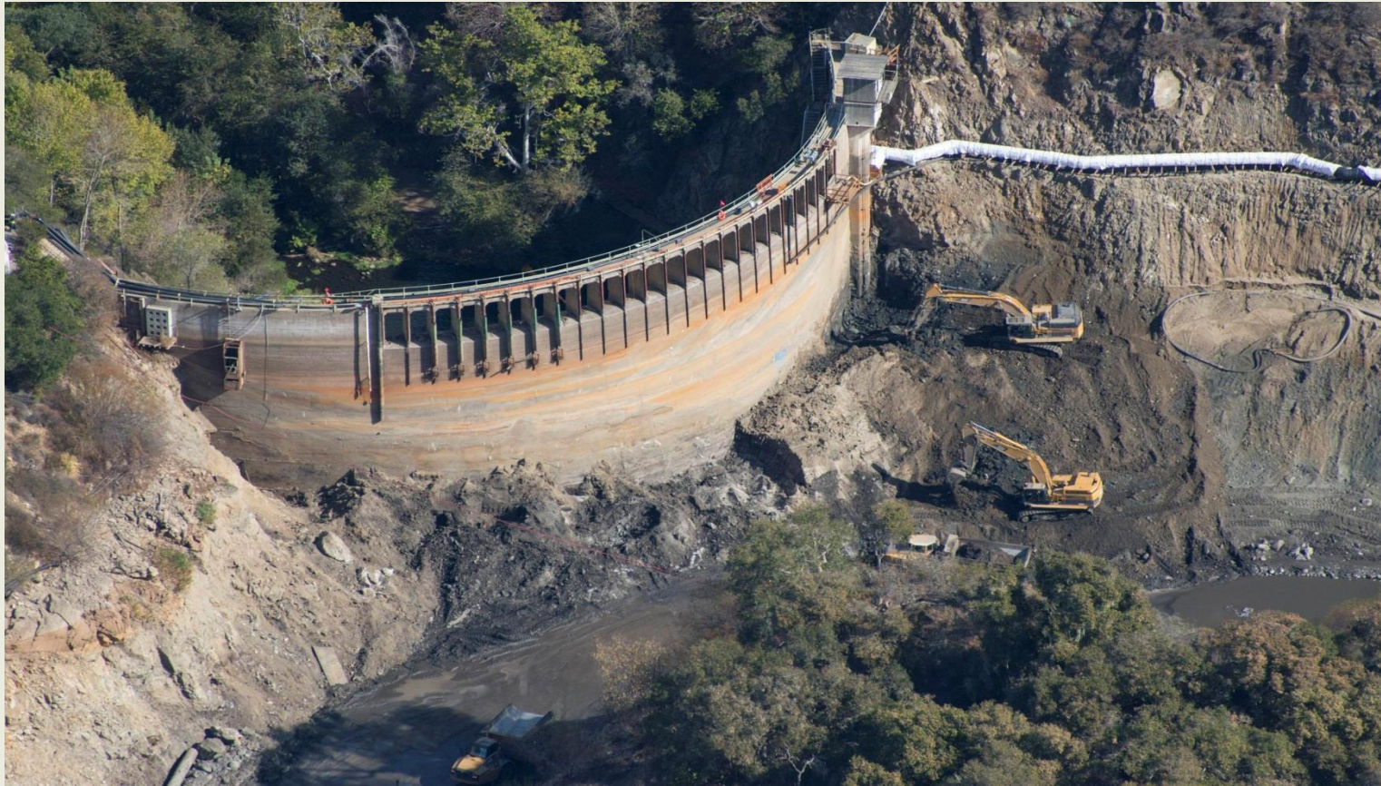
Excavation at bottom of CFR and dam
