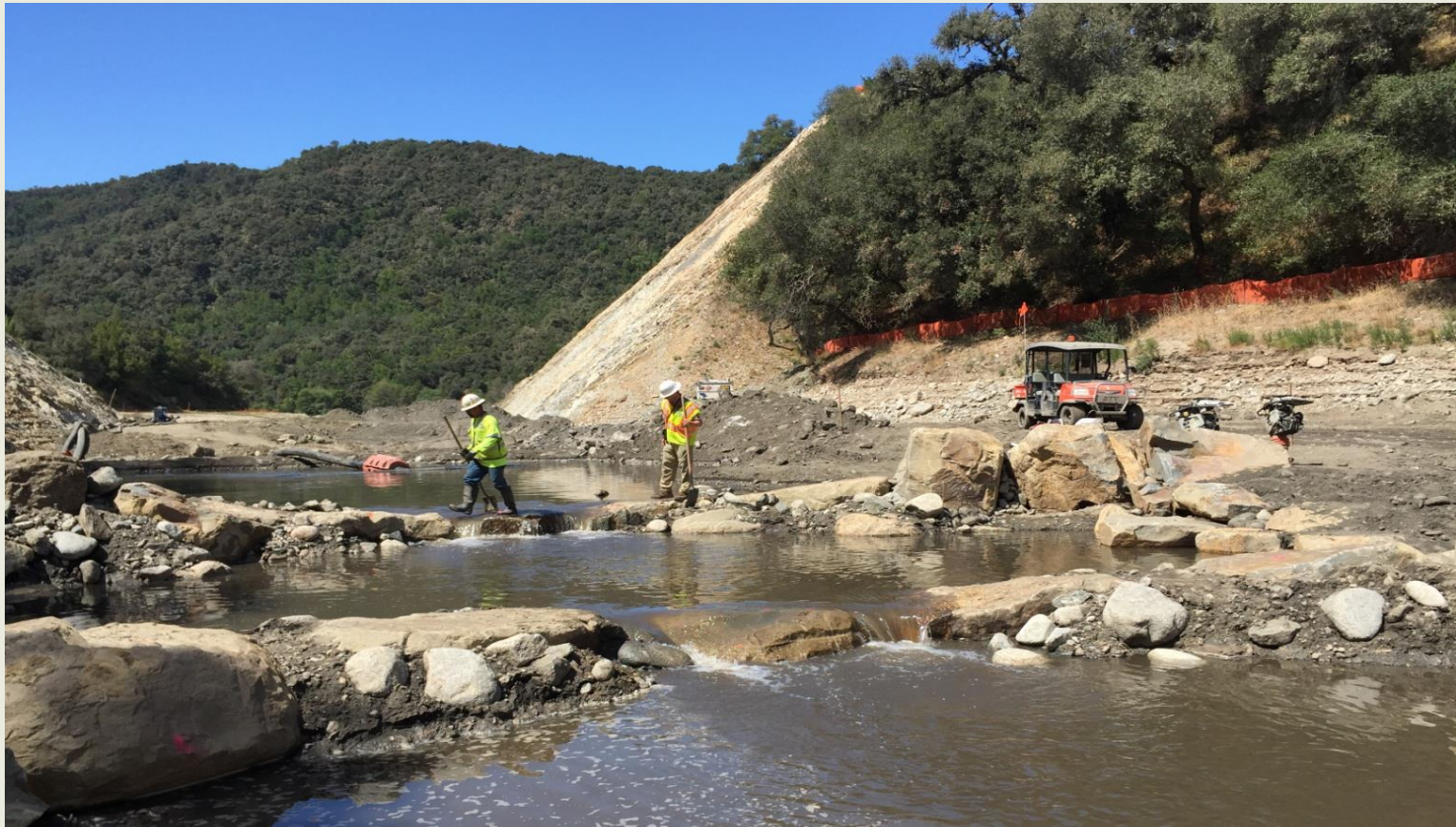
Construction of step pools for channel restoration
