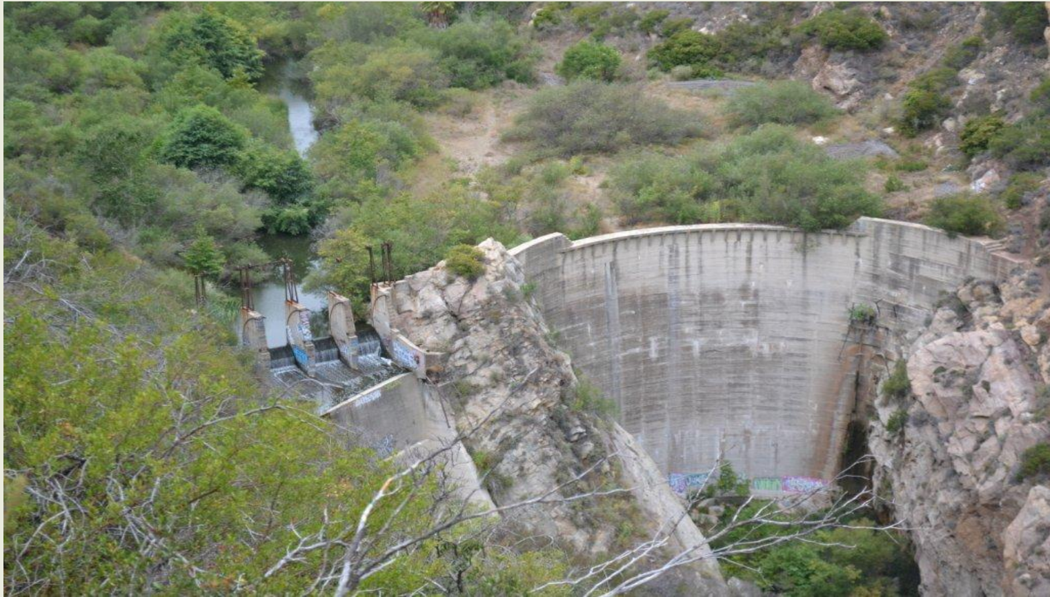
Rindge Dam spillway. Reservoir is completely filled with sediment
