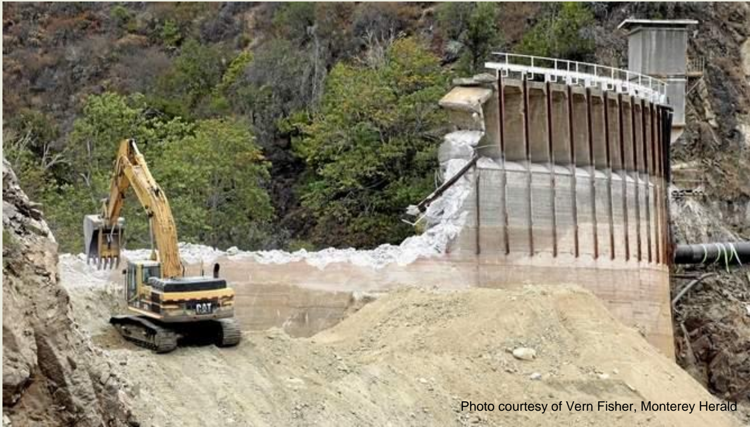
San Clemente Dam demolition underway
