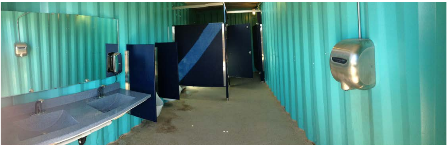
Photograph 2: Panoramic view of the men's restroom showing the paintwork, new partitions, new hand dryer, two new urinal stalls, double basin sink, automatic soap dispenser, and epoxy flooring (AFTER PROJECT). (Photo by K.C. O'Shea)
