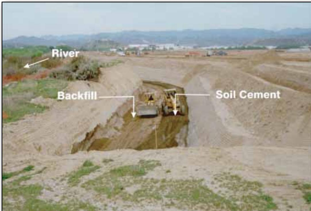
**Buried Soil Cement Backfill**
