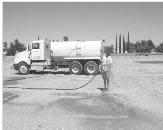
Figure 2-2: Topical application of a dust suppressant using a spray hose.
