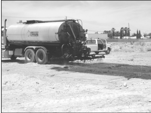
Figure 2-3: Topical application of a dust suppressant using a spray bar.
