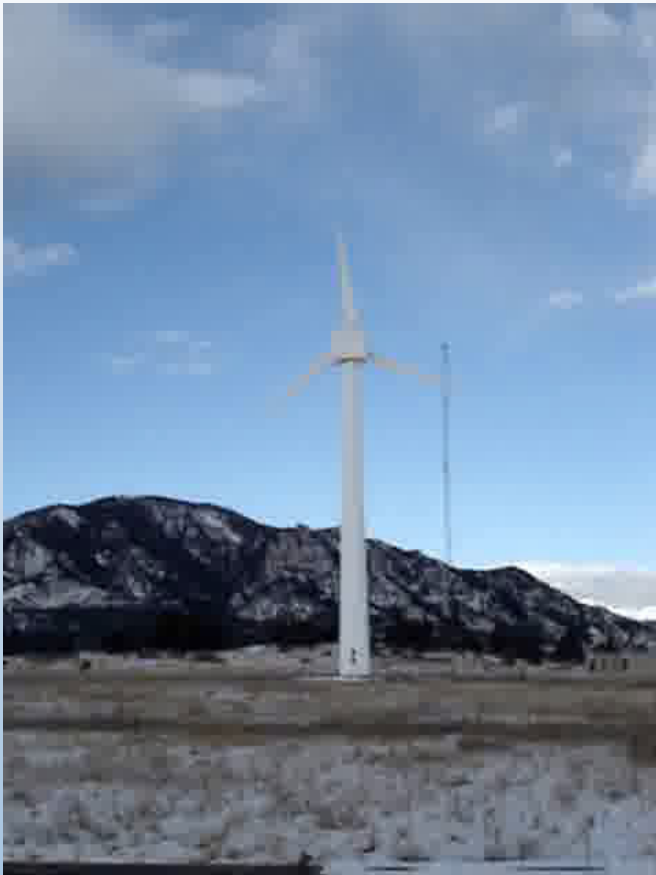
15 Meter Diameter and 100 kW
