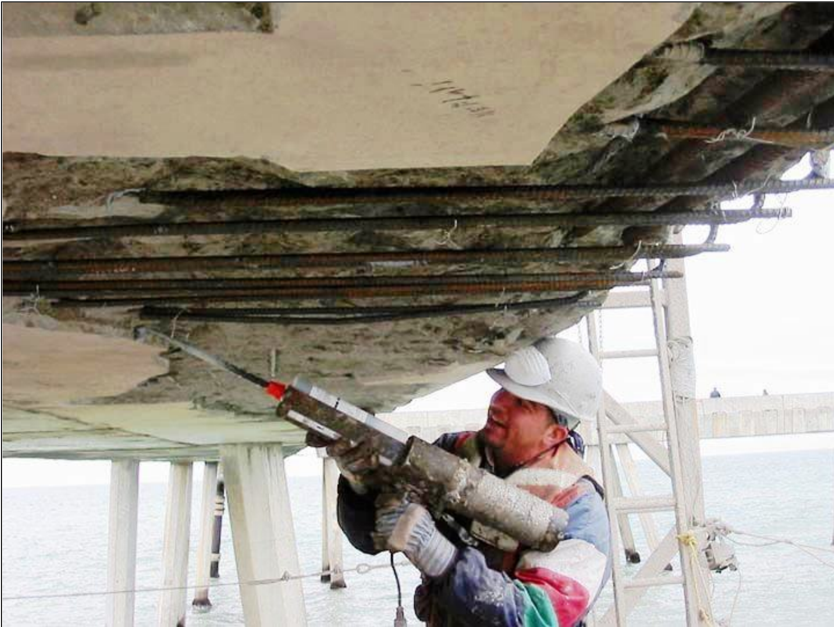
Image 10: Example of repair techniques on other piers (3 of 3). Presented to assist with cost estimating discussions.
