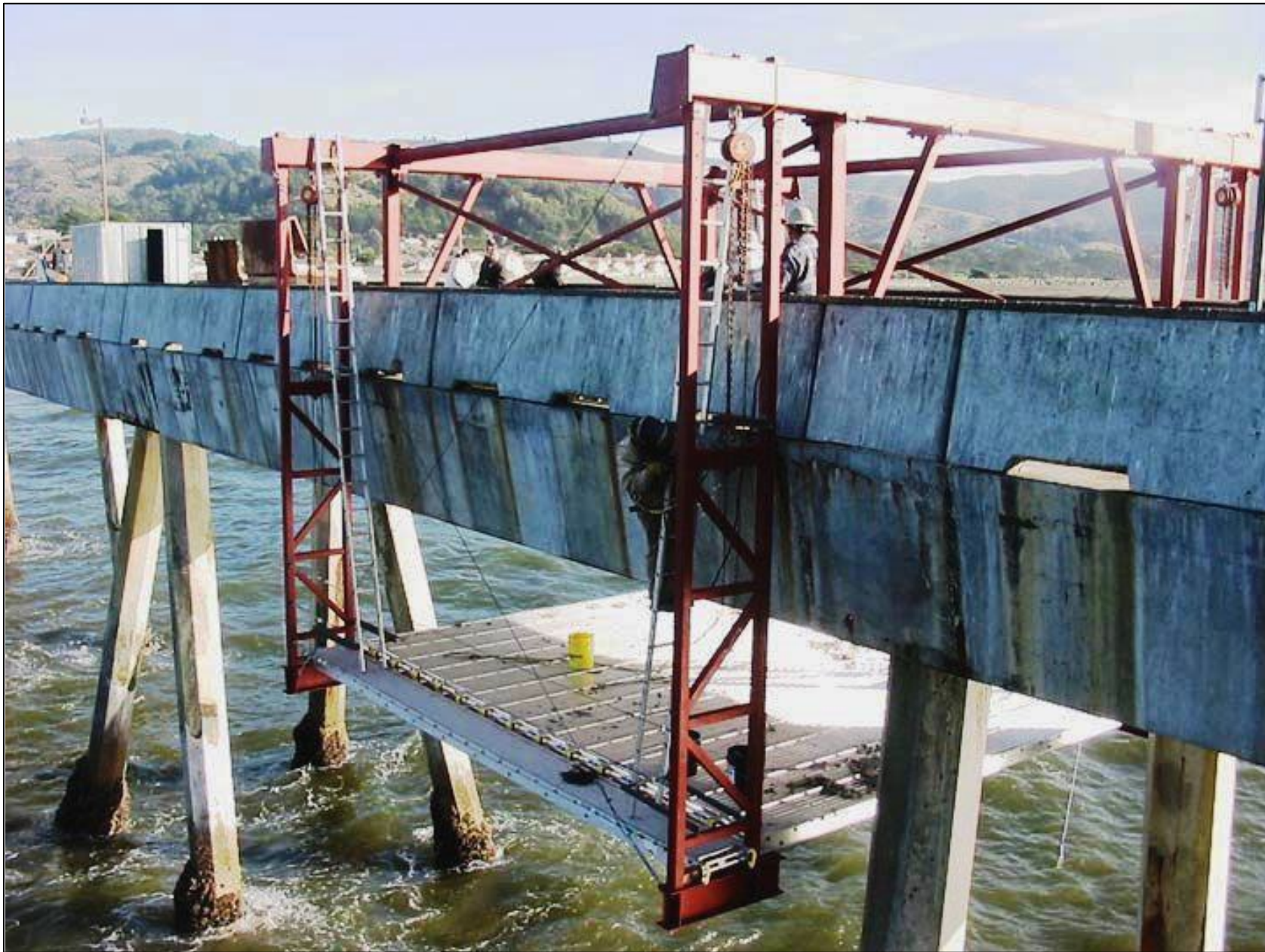
Image 8: Example of repair techniques on other piers (1 of 3). Presented to assist with cost estimating discussions.
