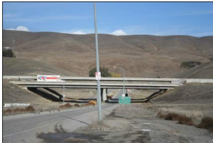
Figure 42: Highway 101 Golf Course Drive Underpass.
