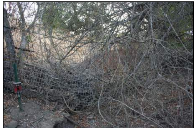
Figure 17: Fencing on south side of Bailey Bridge.
