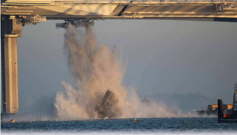
Staff wrote an incidental take permit amendment that would ensure the environmental effects from the implosion of pier E3 (San Francisco Bay Bridge) were monitored and that appropriate mitigation actions were identified.
