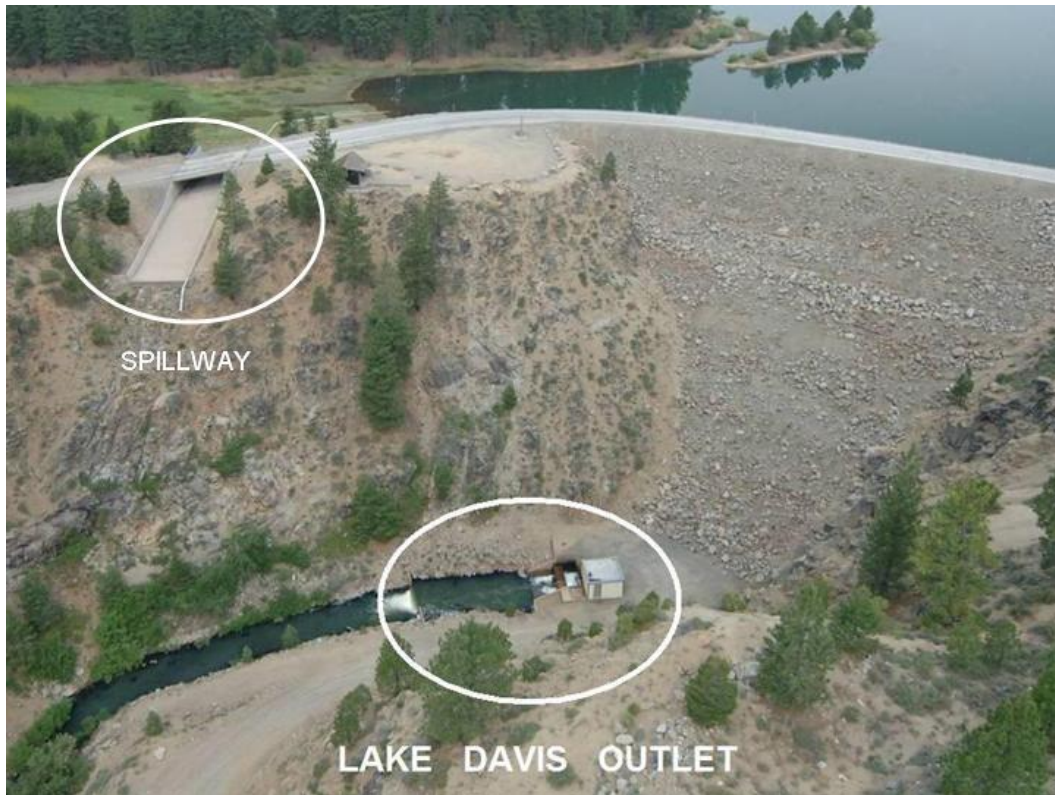
Figure 1. Lake Davis showing Grizzly Valley Dam, the spillway, and outlet structure (pre-fish containment structure).
