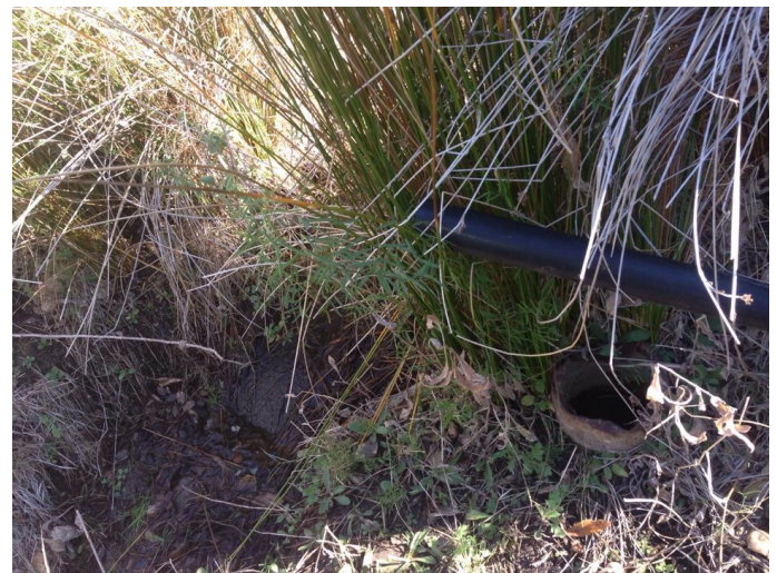
The extended fill pipe no longer serving its purpose.
