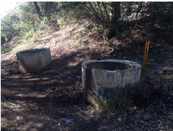
The current concrete troughs that attempt to retain the spring water.
