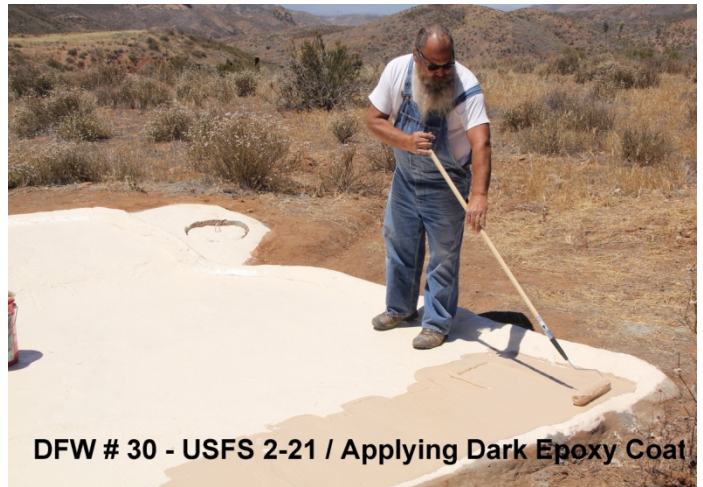
DFW #30 - USFS 2-21 / Sealer & 1st Epoxy Coat Applied
