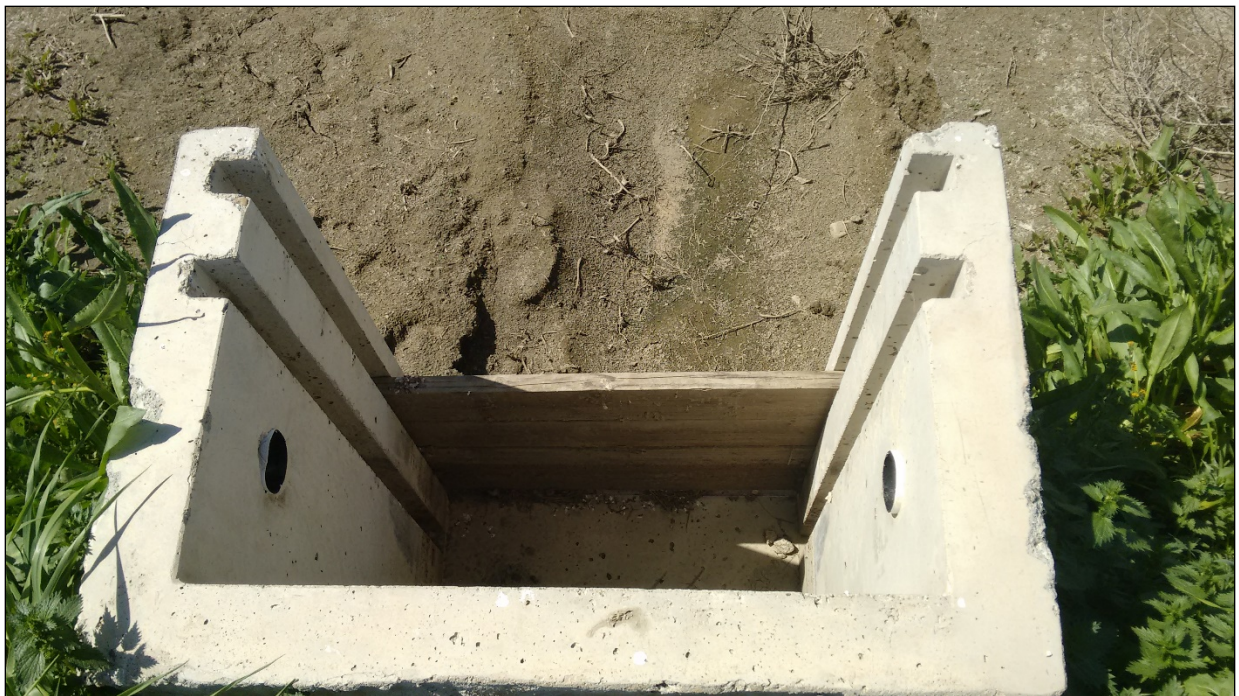
Figure 3. One of five concrete flashboard water control boxes installed at Site 1.
