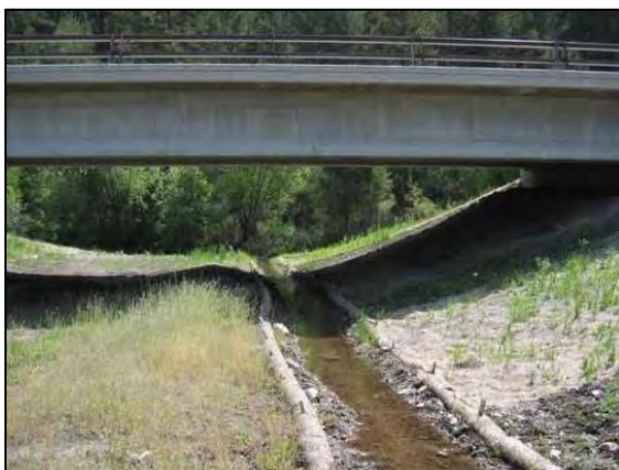
Figure C-3a—Bridge with channel that allows water to flow seasonally.
