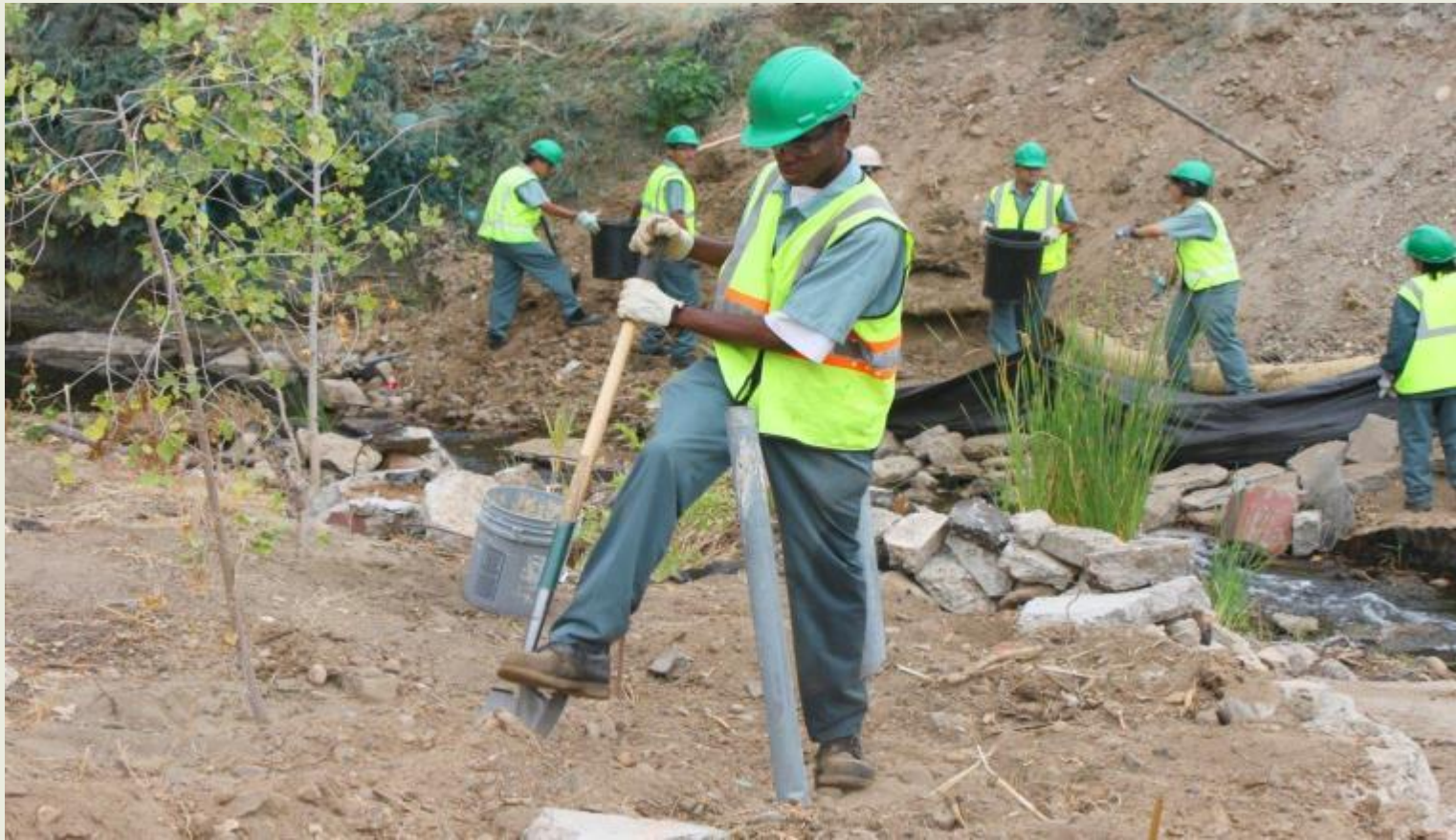
Erosion control & native plant installation – Urban Corps
