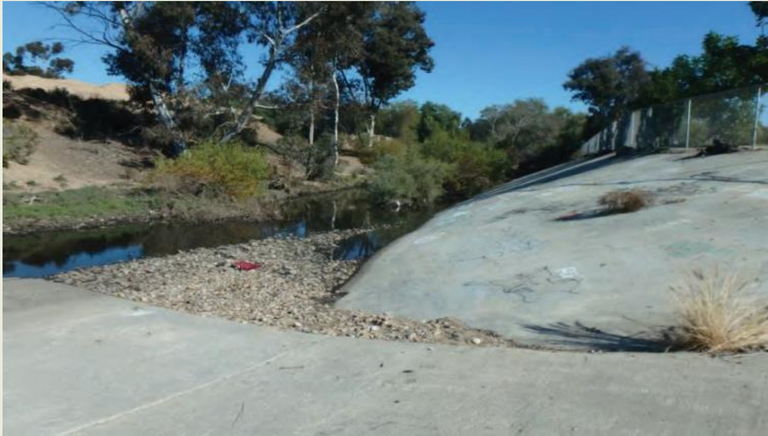
Flood Channel with concrete bank – south bank
