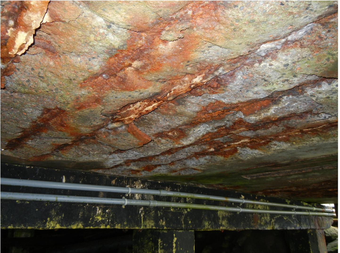
Image 15: A detailed photo of the rusted and snapped structural rebar on the underside of the concrete deck surface of the Pier. An independent structural engineering evaluation found that most of the structural rebar has snapped, leaving the Pier with zero strength to hold up the concrete deck surface, which required the City to close the Pier to public access. (Photo Credit: Roger Miller)
