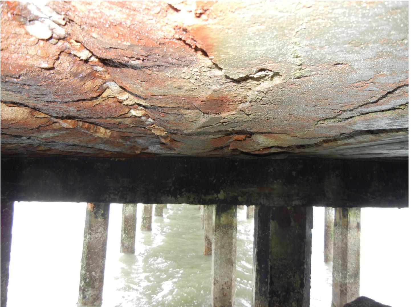
Image 14: On the underside of the concrete deck surface of the Pier, the bottom layer of concrete has spalled off, exposing the structural rebar, which has snapped and failed for the most part, throughout the entire length of the 3,000 foot Pier. On the upper right, see the partially remaining layer of concrete that was applied to the underside in 1984, to prolong the life of the structural rebar. (Photo Credit: Roger Miller)
